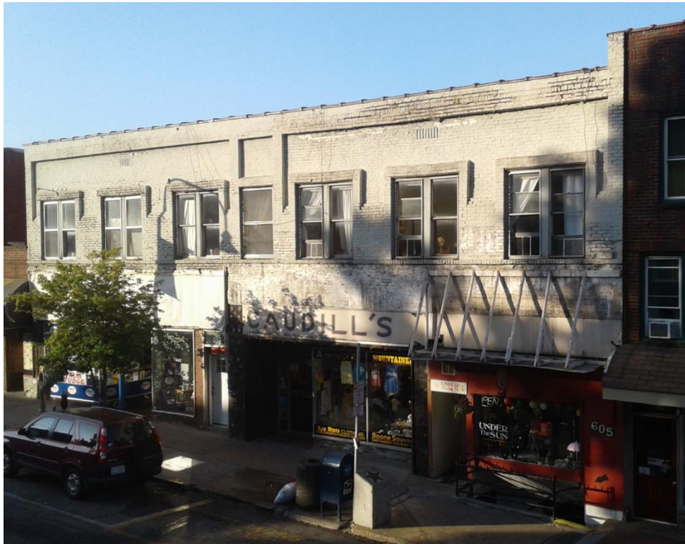
Graphic 14.19.06-3 Desired Downtown Design: 607 West King Street Identified Features: Original brick materials, brick detailing and coping; fenestration percentages; transom over door
