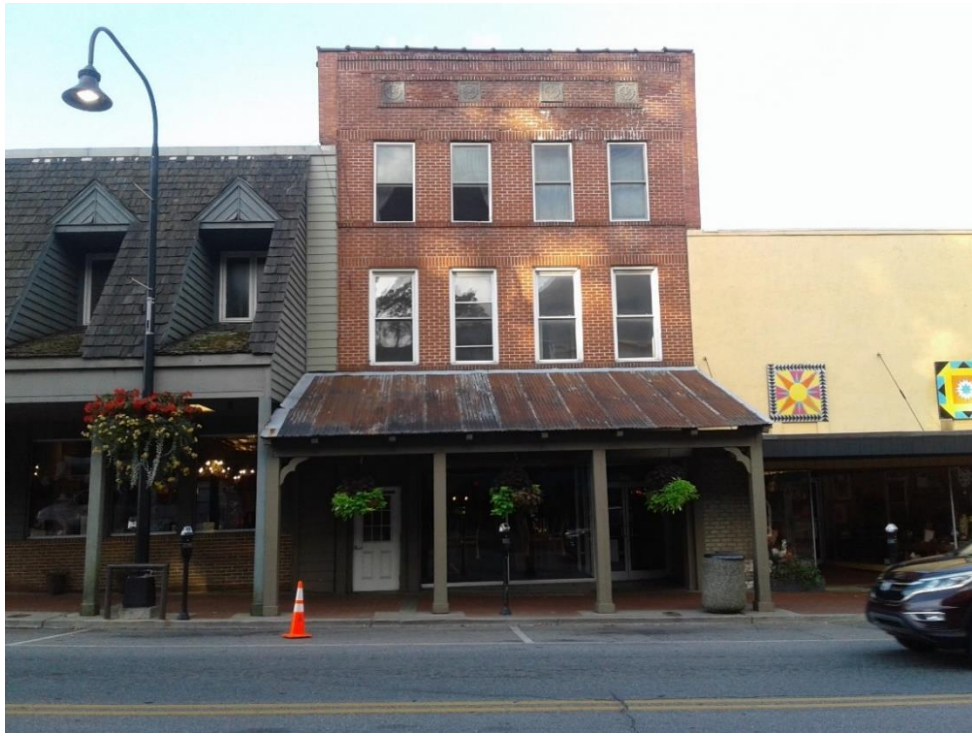
Graphic 14.19.06-5 Desired Downtown Design 630 West King Street Identified Features: Original brick materials, brick detailing; fenestration percentages; clerestory windows; doors; storefront window; awnings
