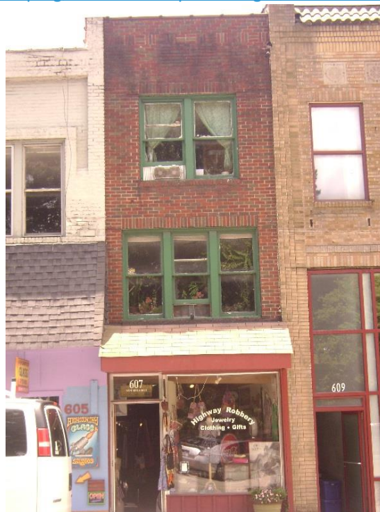
Graphic 14.19.06-3 Desired Downtown Design: 607 West King Street Identified Features: Original brick materials, brick detailing and coping; fenestration percentages; transom over door
