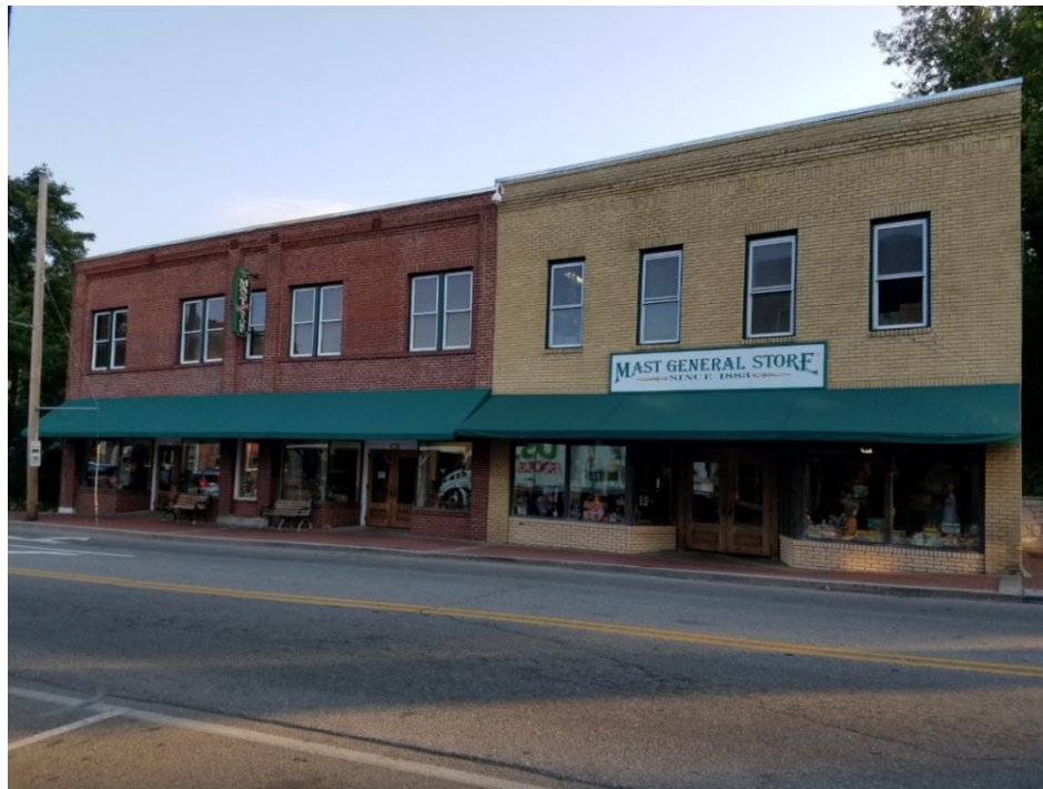
Graphic 14.19.06-5 Desired Downtown Design 630 West King Street Identified Features: Original brick materials, brick detailing; fenestration percentages; clerestory windows; doors; storefront window; awnings
