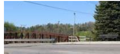
Existing Site Conditions
