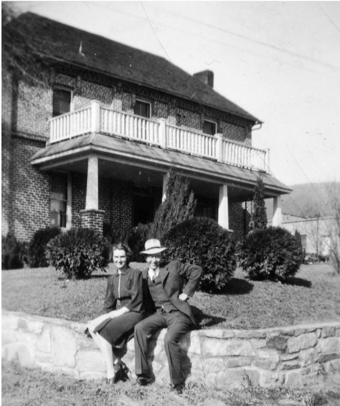
Detail crop showing Louise Wyke Russell (L) and an unidentified man sitting on the stone wall in front of the Watauga County Jail building during the 1930s. Image courtesy of the David Wyke Collection, Digital Watauga Project.
