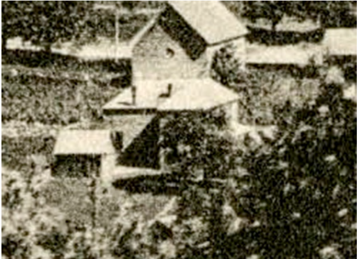
Detail crop from a 1915 postcard showing the south and east elevations of the Watauga County Jail from the southeast. A hipped-roof porch clearly appears to be visible projecting from the east elevation of the jail, confirming the presence of a front porch as early as 1915. Image courtesy of the Bobby Brendell Postcard Collection, Digital Watauga Project.
