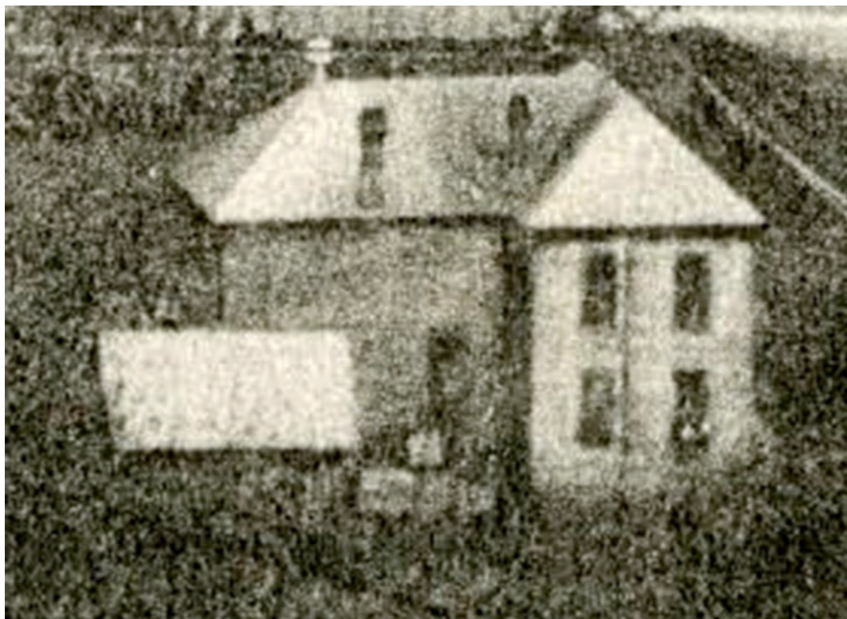
Detail crop from a 1905 postcard showing the south elevation of the Watauga County Jail from the southwest. A shed-style, angled bracket appears to be visible projecting from the east elevation of the jail, suggesting the presence of a front porch as early as 1905. Image courtesy of the Bobby Brendell Postcard Collection, Digital Watauga Project.
