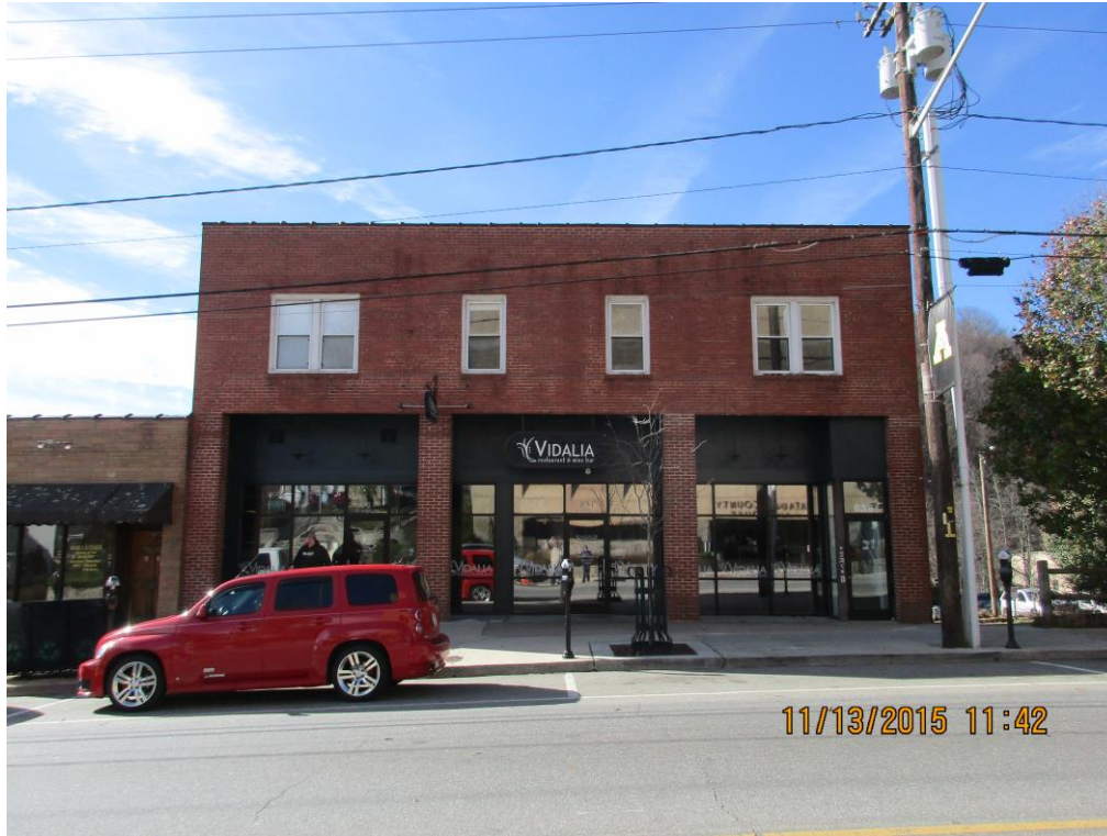
The Edmisten Building as it appeared in November 2015. Image by Eric Plaag.
