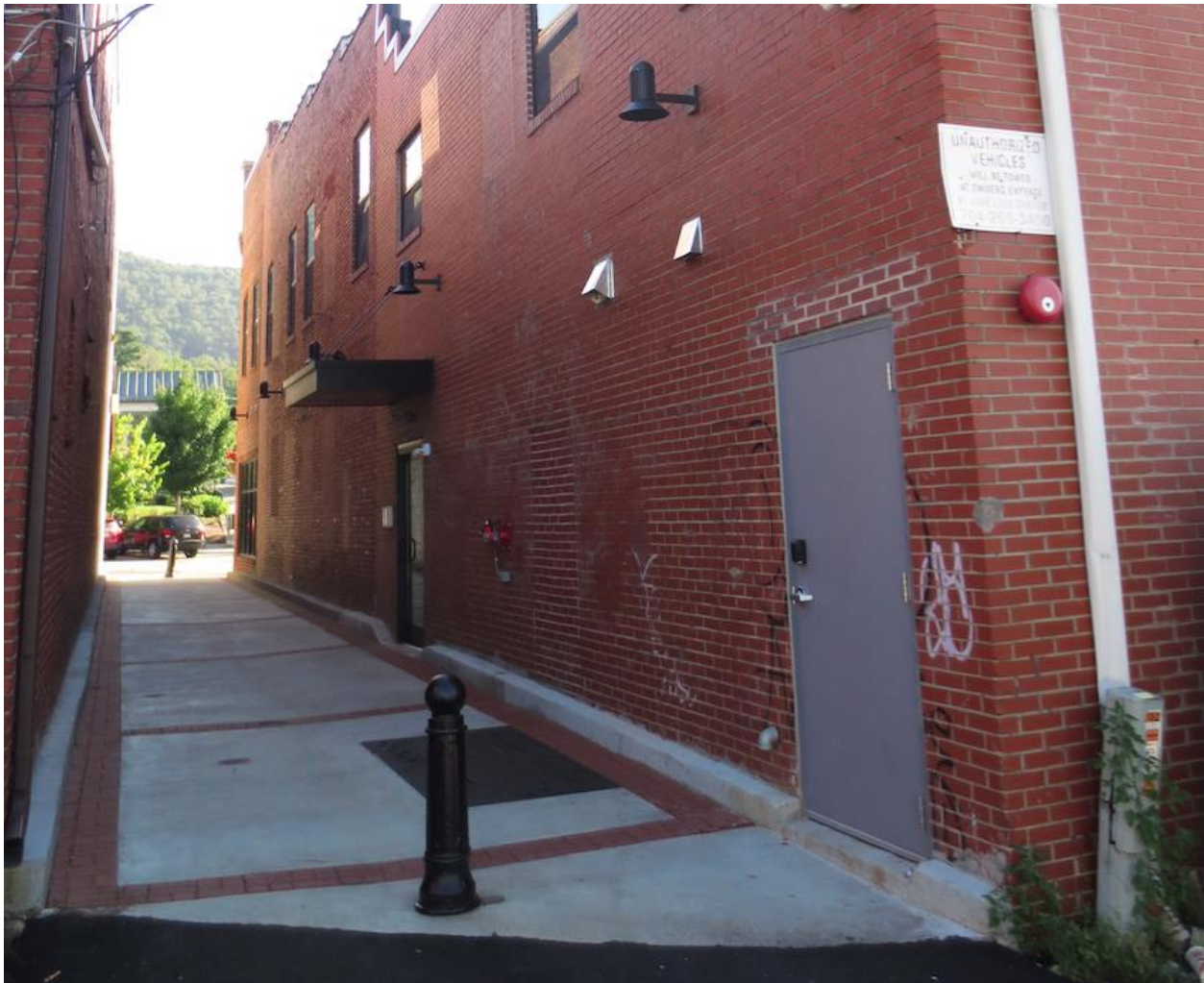
During recent renovations to this King Street property, the architect designed a new but inconspicuous, ADA-accessible fire exit on a secondary elevation adjacent to a public alley, including a curb cut to allow for wheelchair movement. Photo by Eric Plaag, 2019.
