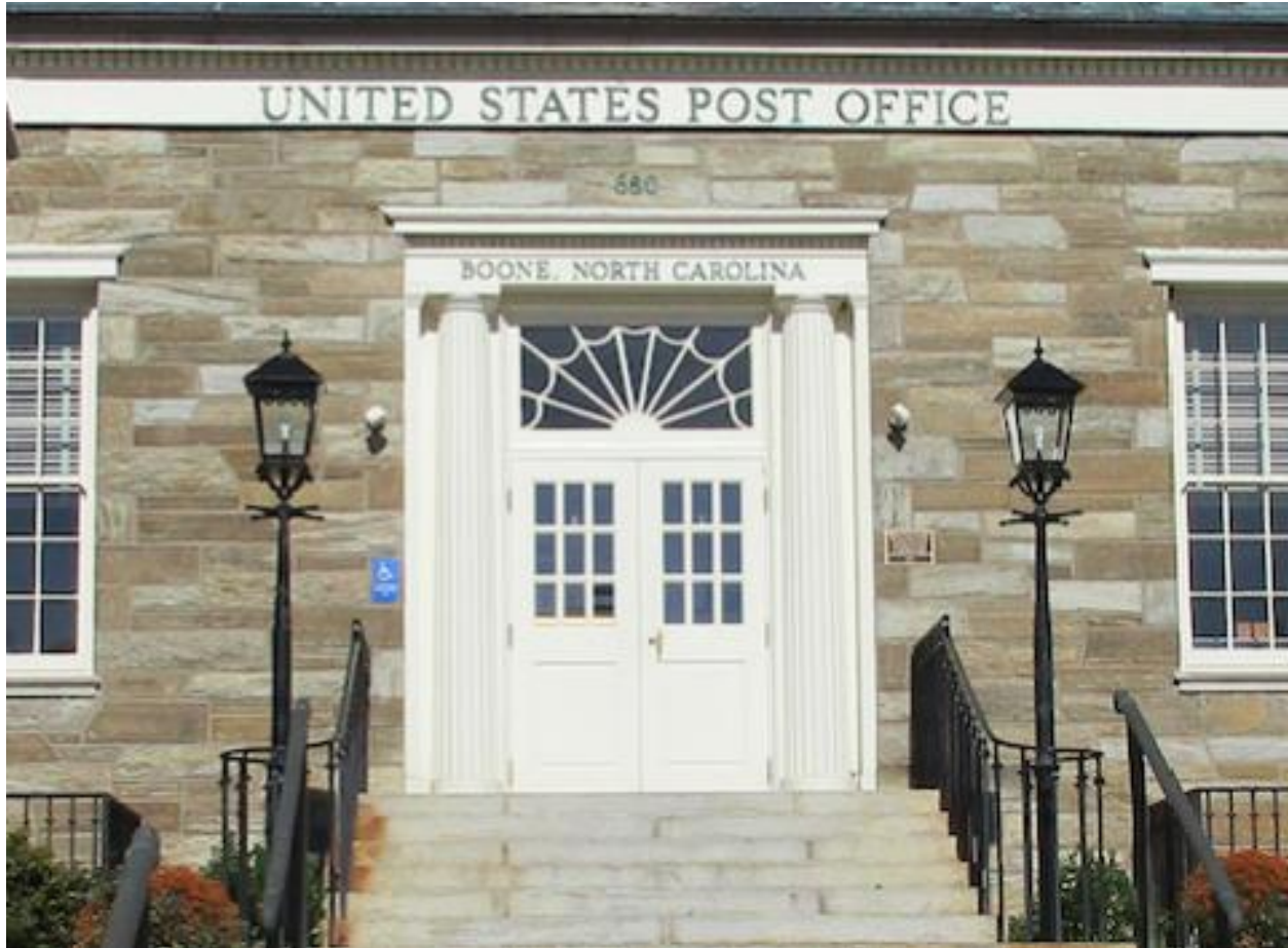
The entrance details of the Boone Post Office are critically important architectural elements for the interpretation and historical integrity of the property, as they help to identify the style of the building as well as its period of construction. Photo by Eric Plaag, 2015.
