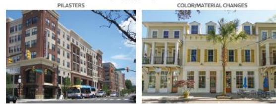
Figure 5.7.E(3)b: Façade Massing
