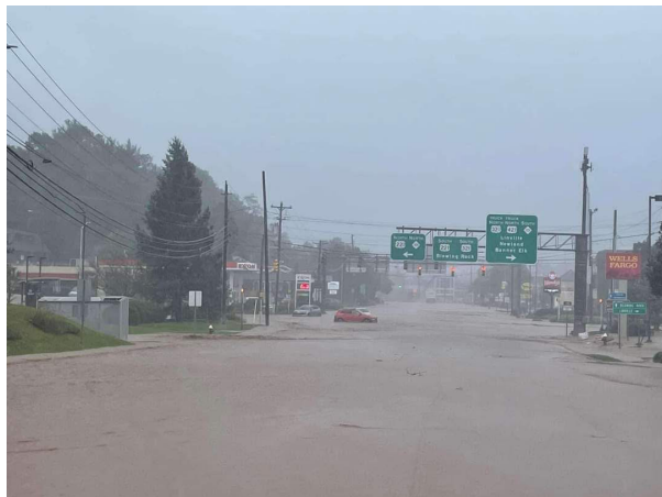
Flooding along Blowing Rock Road in 2024 from Hurricane Helene
