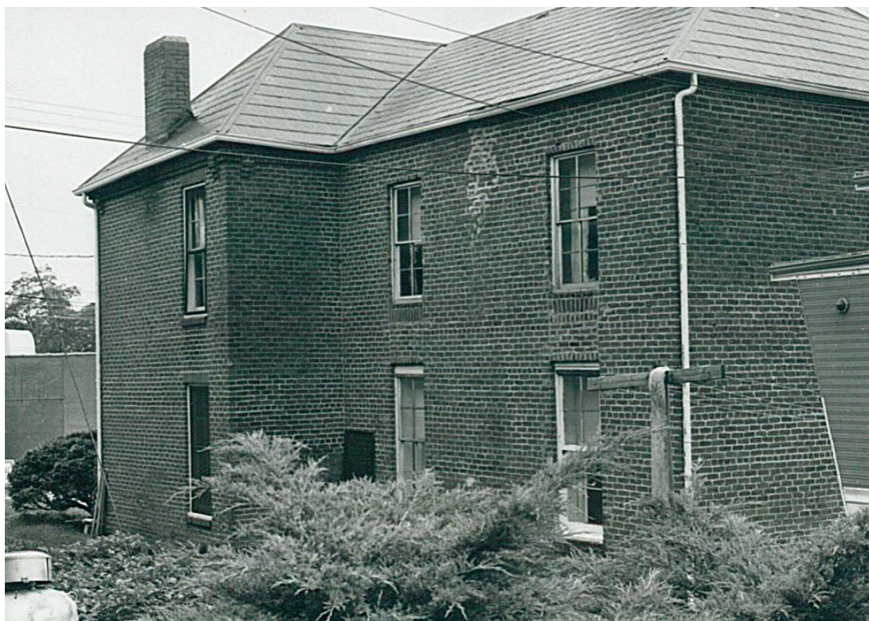
Circa 1982 survey image showing the north elevation prior to the addition of the steel balcony and staircase, with both northwest corner windows intact. Image courtesy of the NC SHPO.
