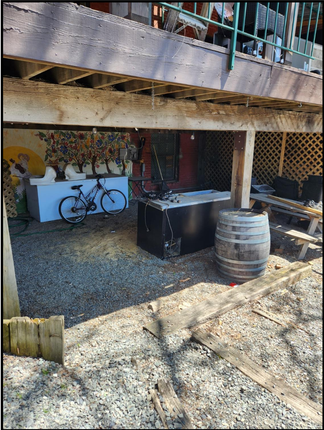
Figure 8: SEBB Under deck area – April 18, 2023.
