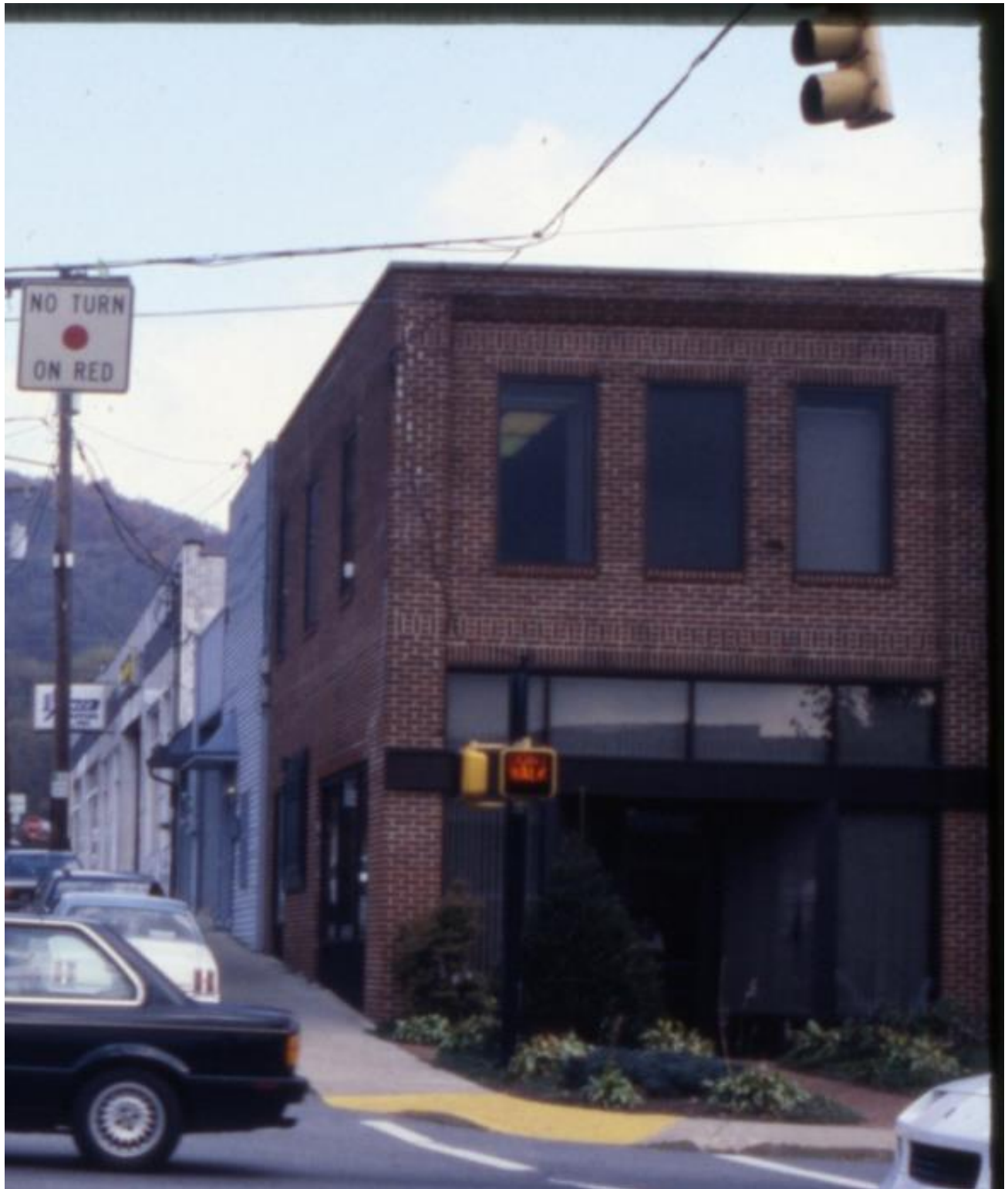
Figure 4. Unknown, "Intersection at King Street and Depot Street, Downtown Boone, 1990s," Digital Watauga, accessed October 26, 2022, https://digitalwatauga.org/items/show/7072 .
