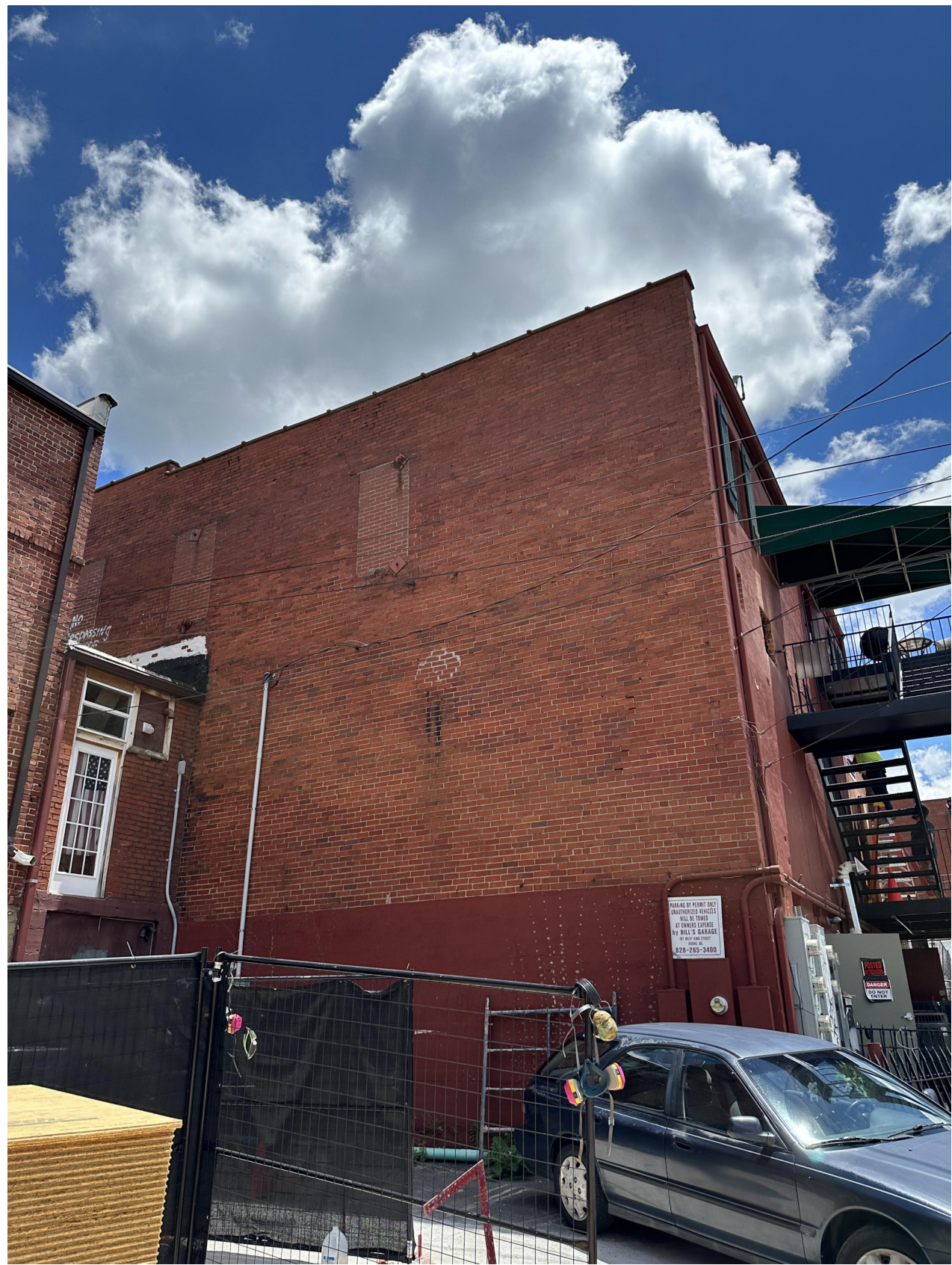
EXISTING BUILDING REAR SIDE
