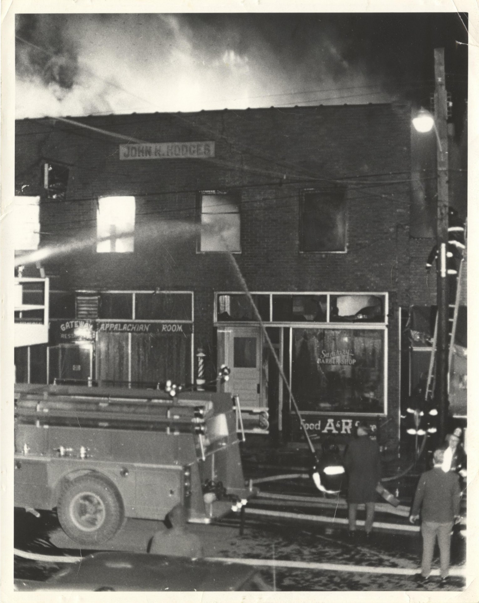
HODGES BUILDING FIRE - 1970, KING STREET FRONTAGE SHOWN
