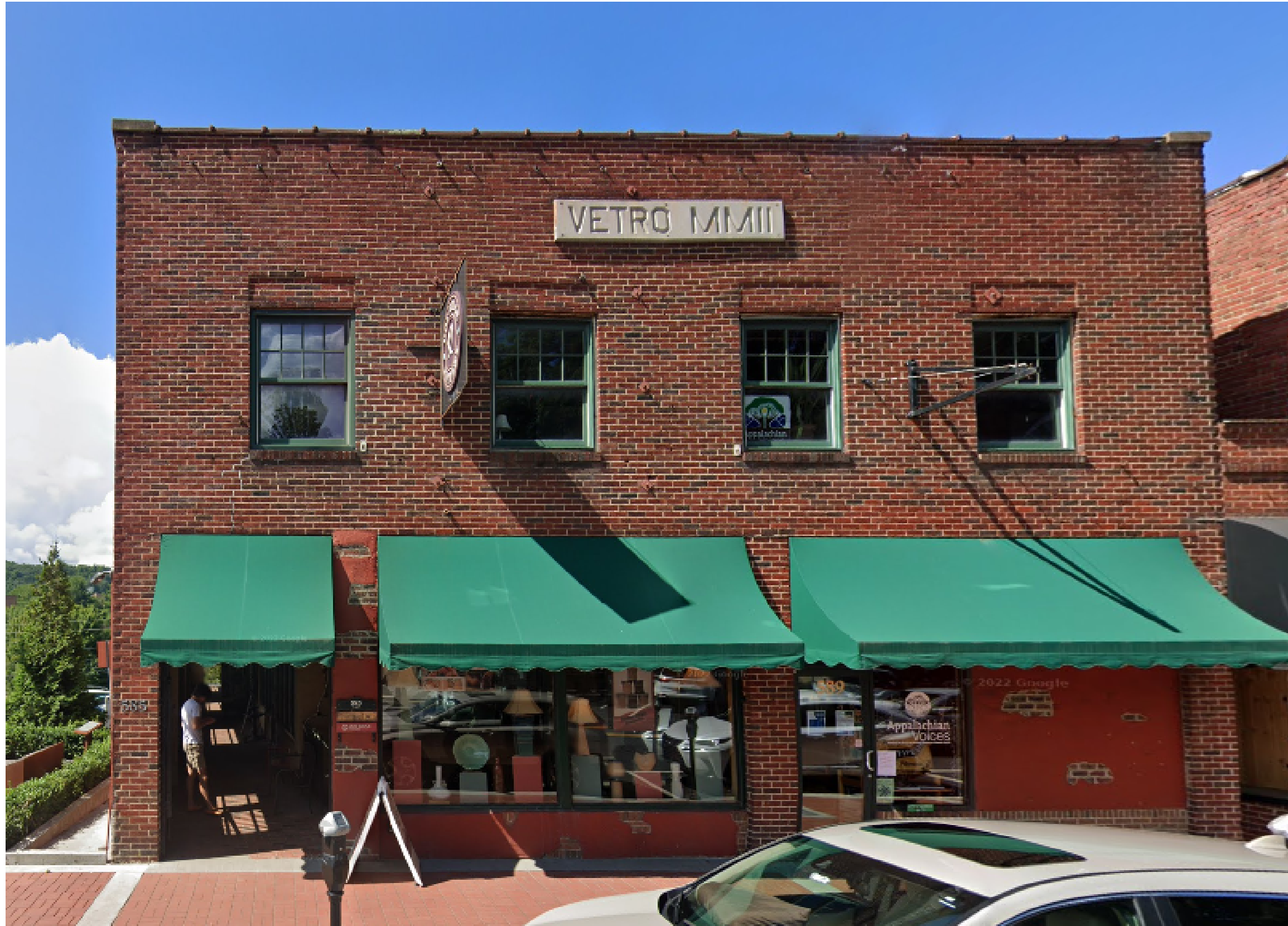
EXISTING BUILDING FRONT
