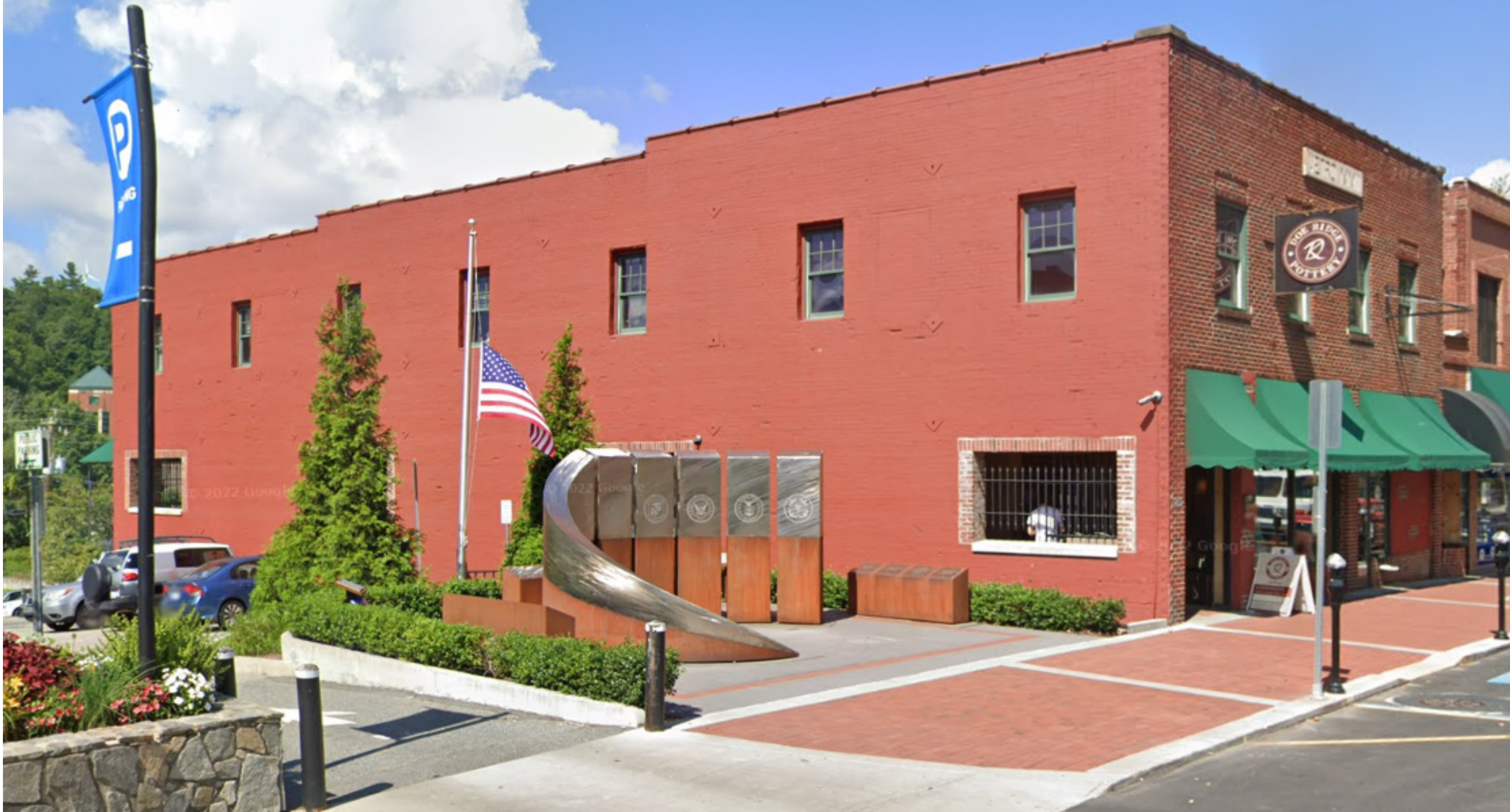
EXISTING BUILDING MEMORIAL SIDE
