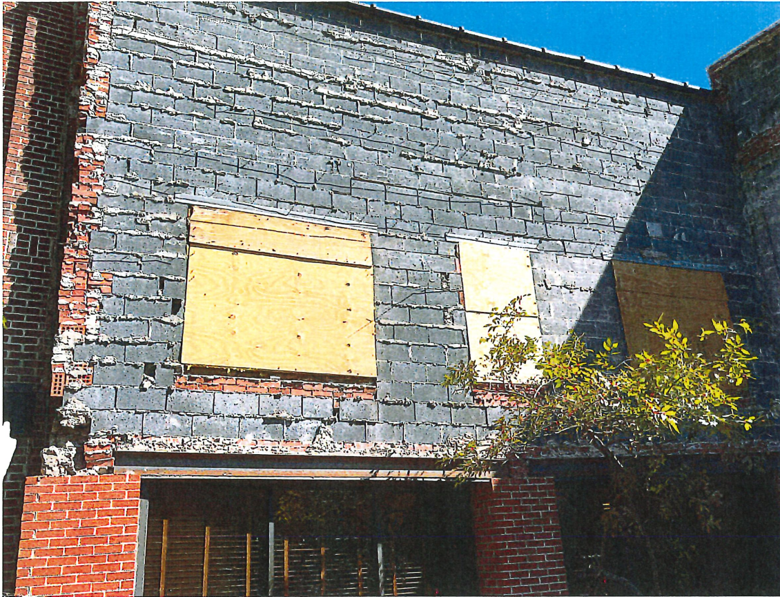
Photographs Illustrating the Current Wall Status
