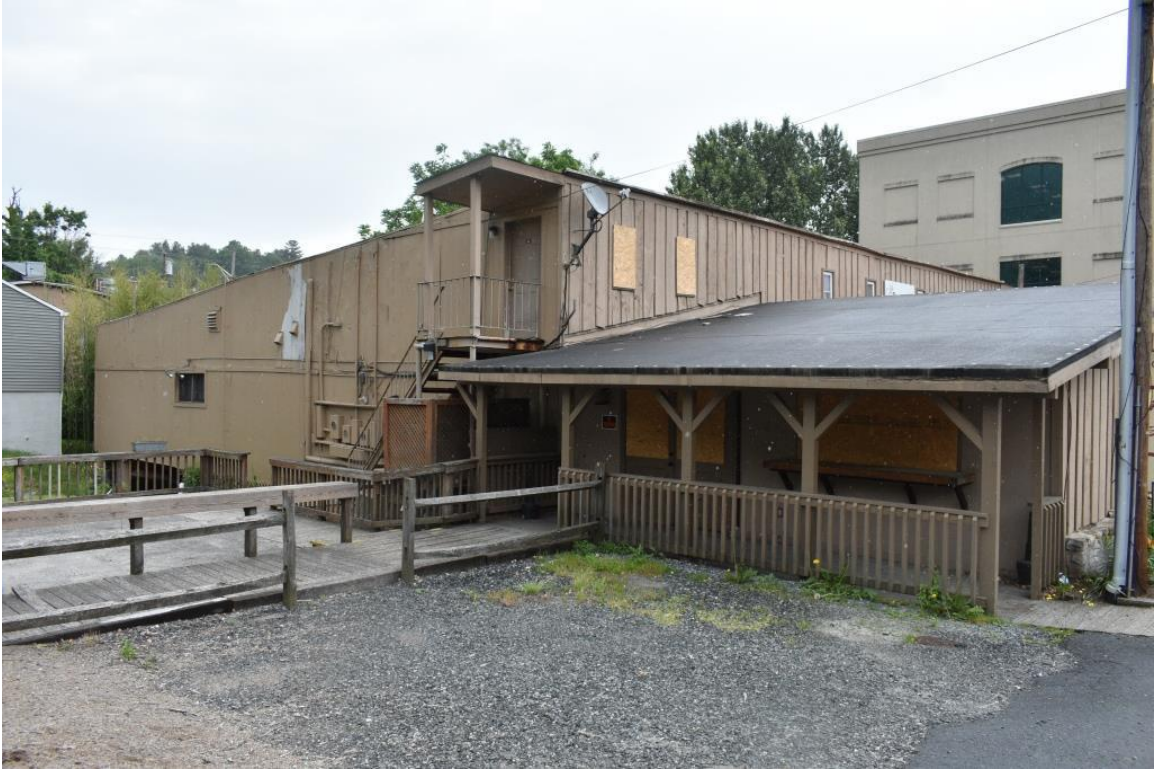
Southwest corner, view to northeast
