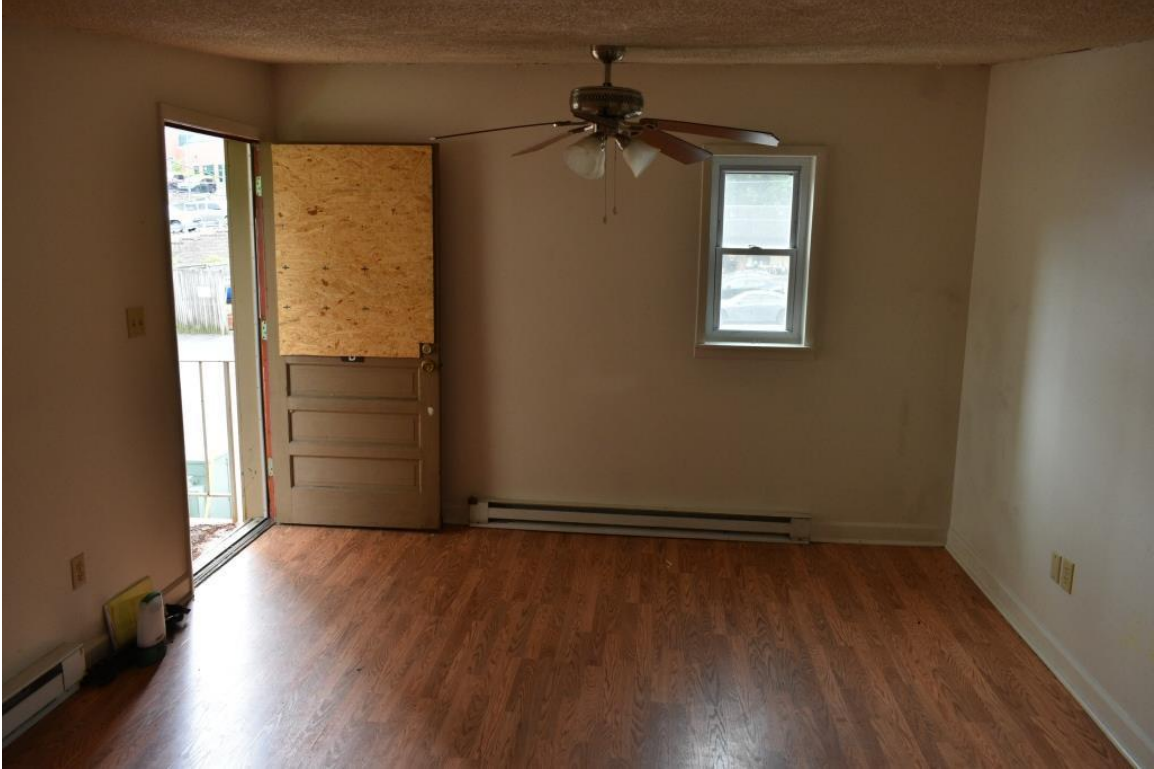
Apartment B, living room, view to southwest
