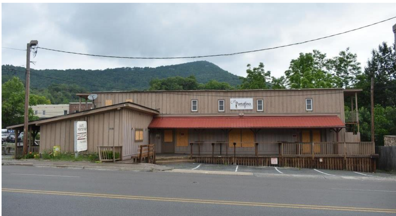
Austin Tobacco Company Prize Room (WT0877), 970 Rivers Street, façade, view to northeast
