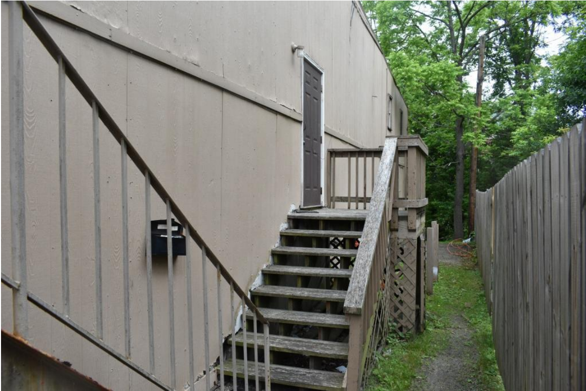
Central entrance door on southeast side elevation, view to north
