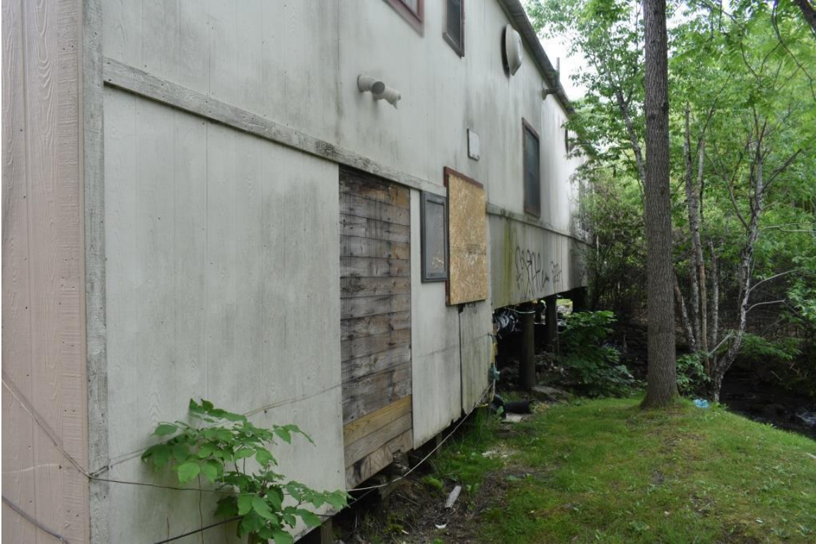
Rear elevation, oblique view to west
