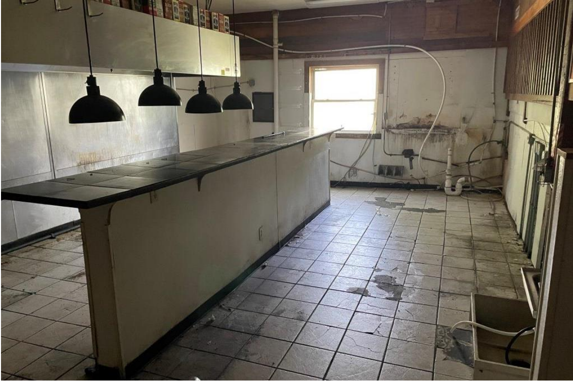
Restaurant kitchen, view to north
