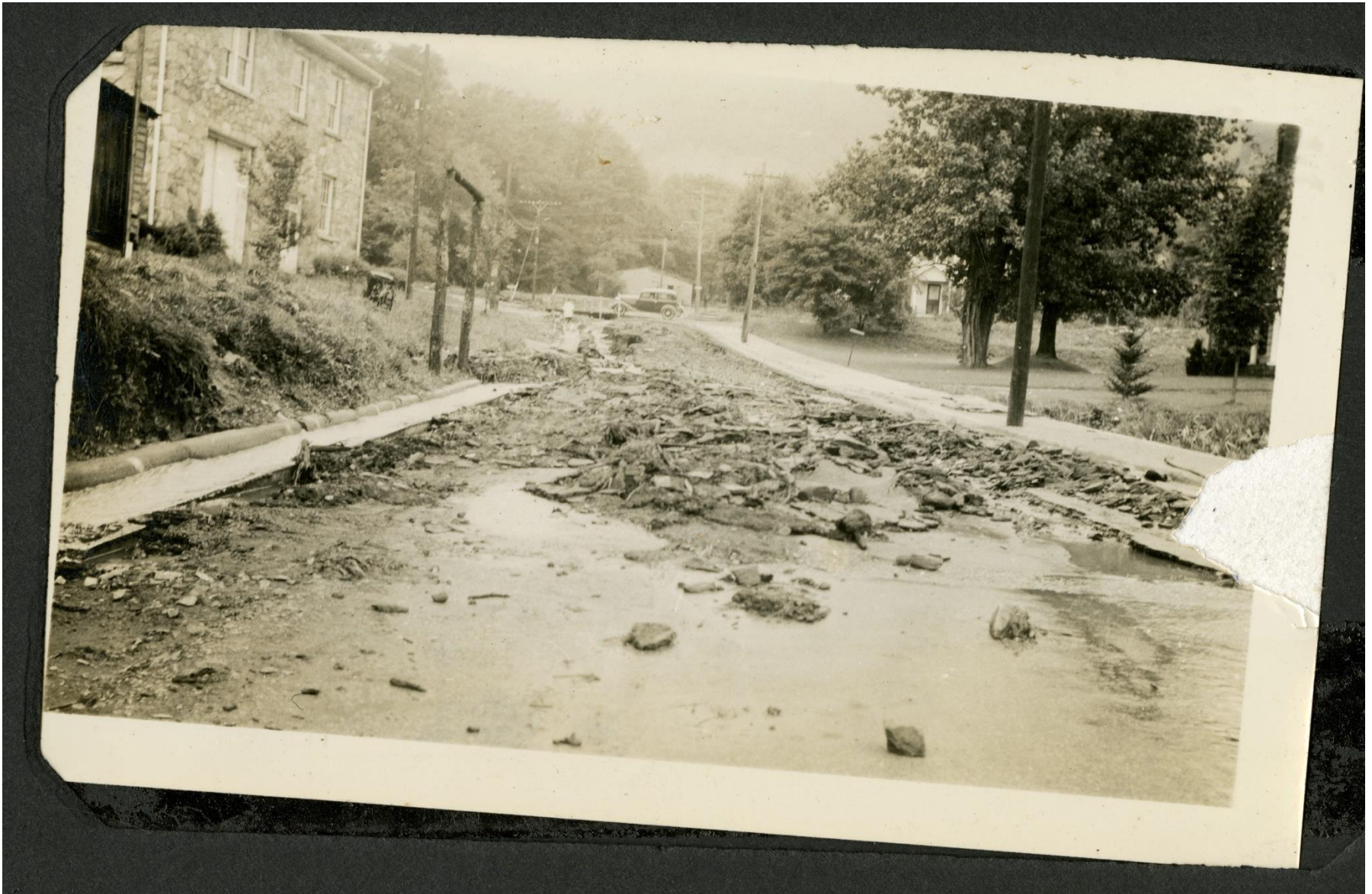
Figure 3. Paul Weston, "Flood Damage, North Water Street #2, Boone, NC, August 1940," Digital Watauga, accessed June 28, 2022, http://digitalwatauga.org/items/show/6345 .
