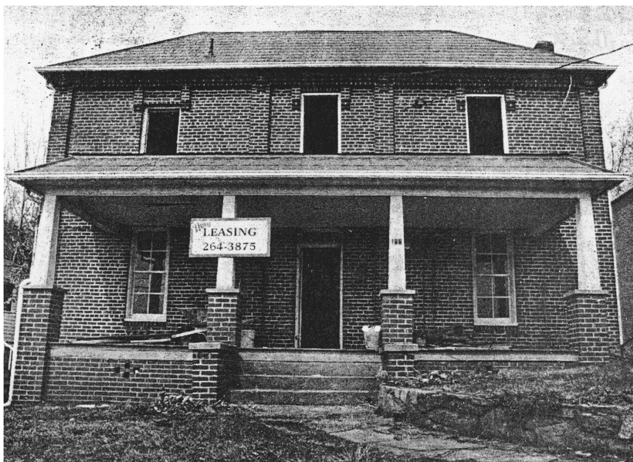
The Watauga County Jail underwent significant renovations in 1985 and 1986 following its acquisition by Don and Mary Dunlap. This image, taken near the completion of renovations, shows the building circa March 1986. Image from the Watauga Democrat , courtesy of the Historic Boone Collection, Digital Watauga Project.
