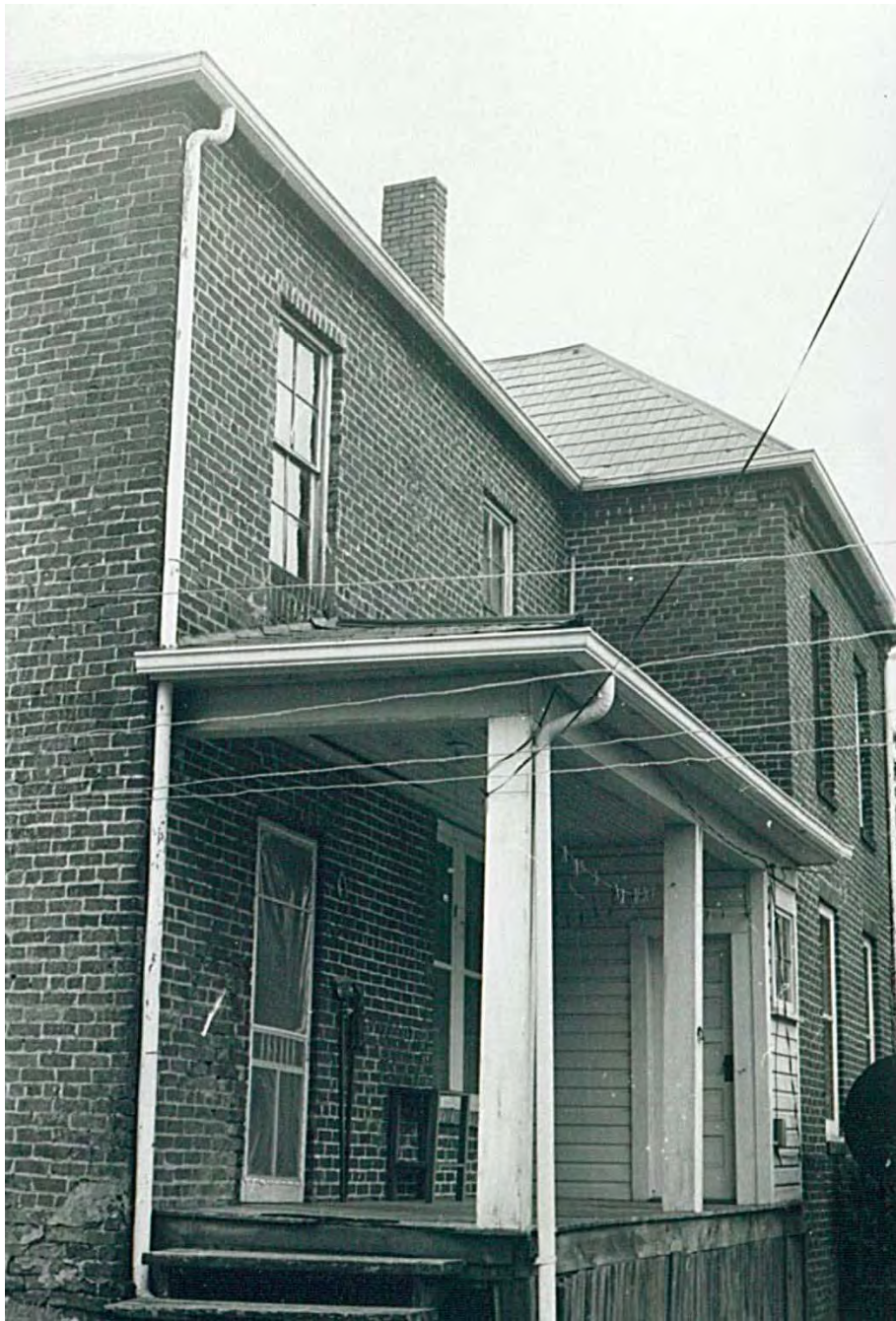
Circa 1982 image showing the south porch prior to its enclosure. Image courtesy of the NC SHPO.
