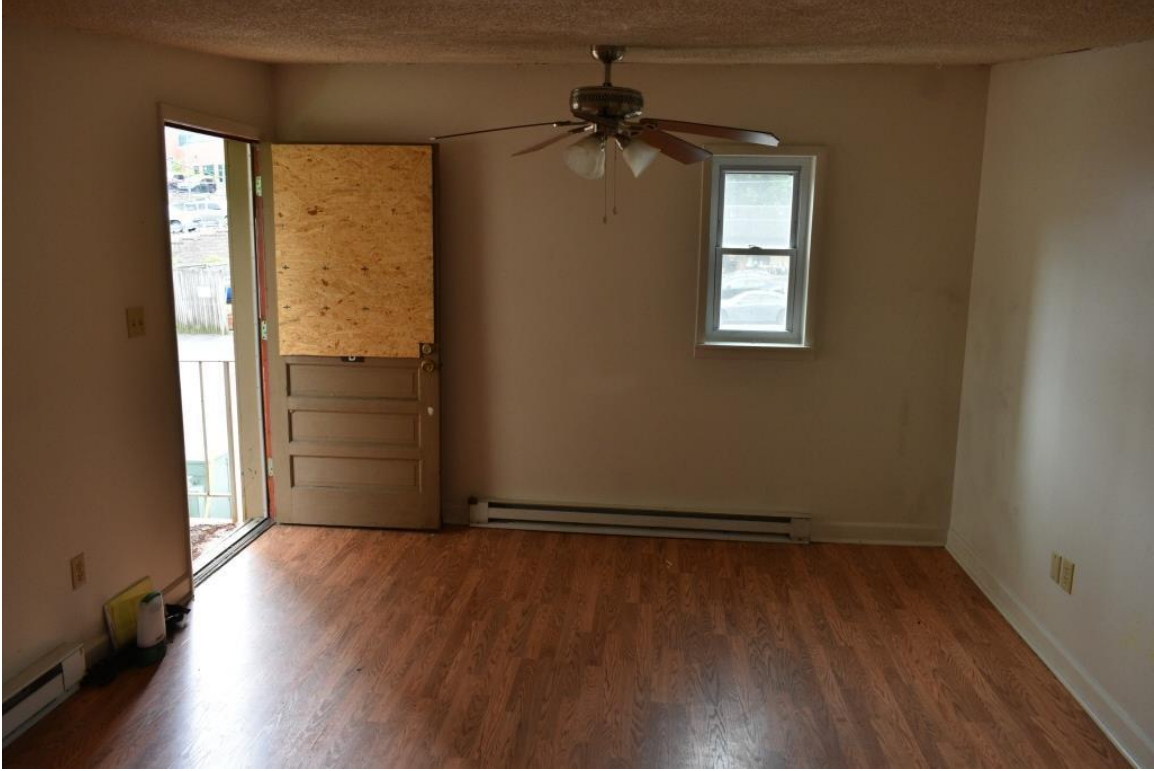
Apartment B, living room, view to southwest
