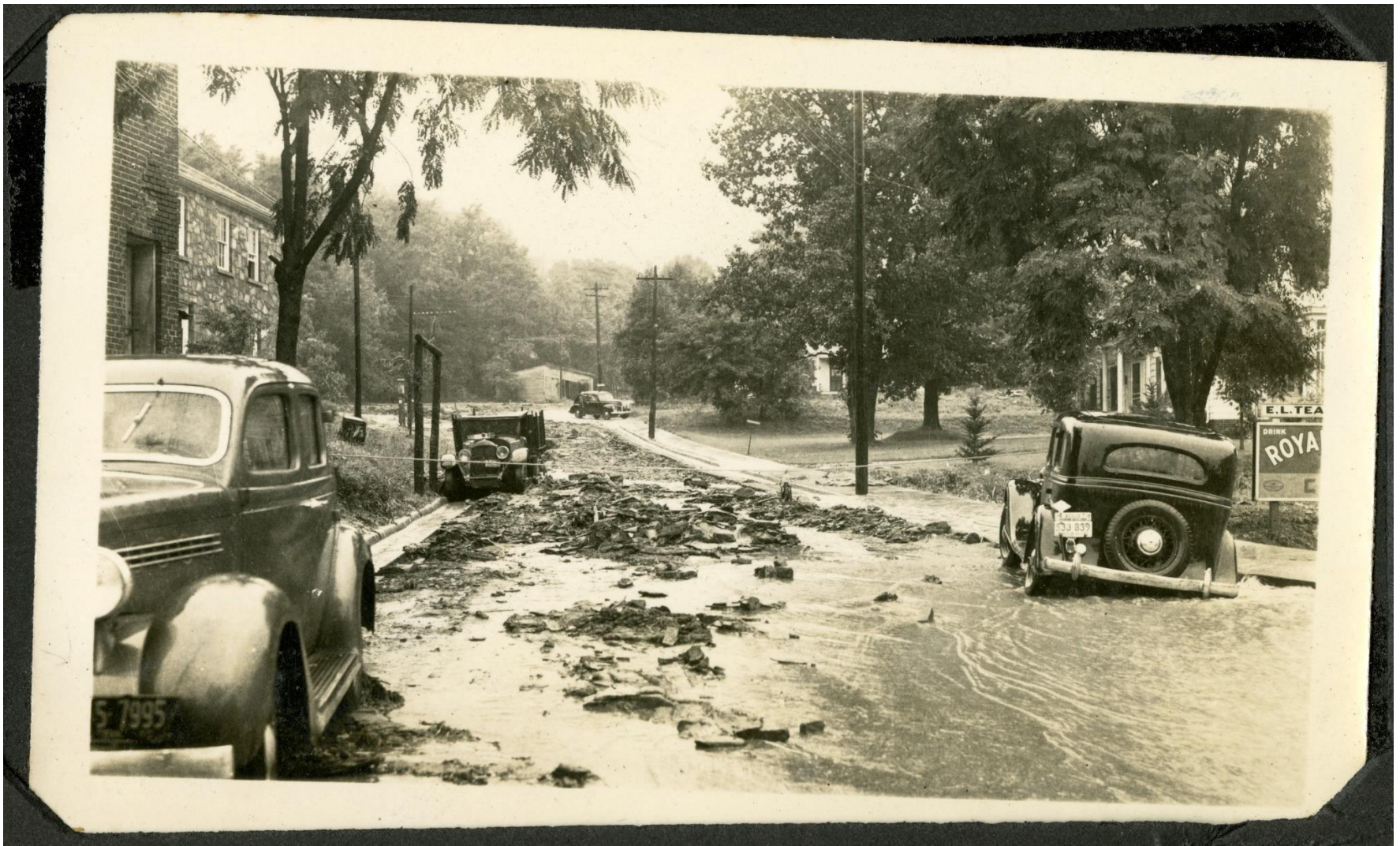
Figure 2. Paul Weston, "Flood Damage, North Water Street, Boone, NC, August 1940," Digital Watauga, accessed June 28, 2022, http://digitalwatauga.org/items/show/6344 .
