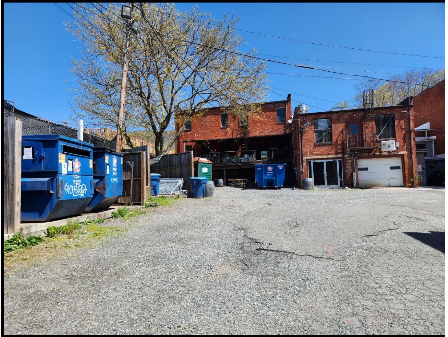
Figure 2: SEBB View from mid-alley way, including proposed area for back patio renovations – April 18, 2023.
