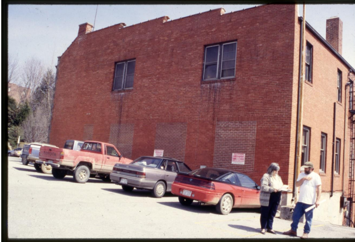
Figure 1: Side View of 747 West King Street in Downtown Boone, April 1996
