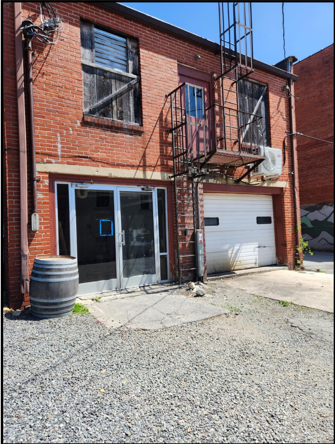
Figure 9: SEBB Back exit to basement and fire escape exit from kitchen (extension of Critcher building) – April 19, 2023
