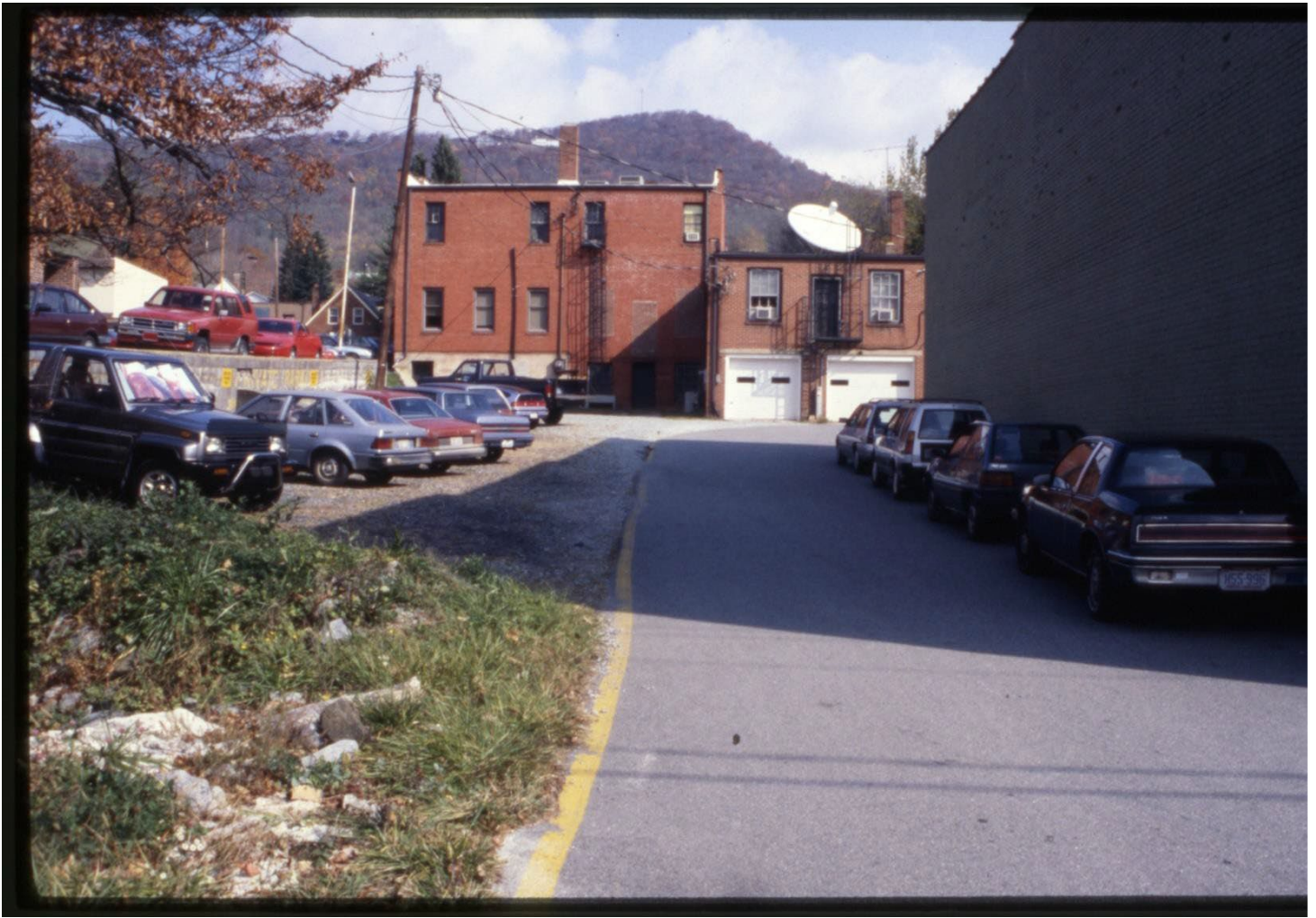
Figure 2. Unknown, "Alleyway and Rear Facades of King Street Buildings, Downtown Boone, 1990s," Digital Watauga, accessed March 30, 2023, https://digitalwatauga.org/items/show/7052 .
