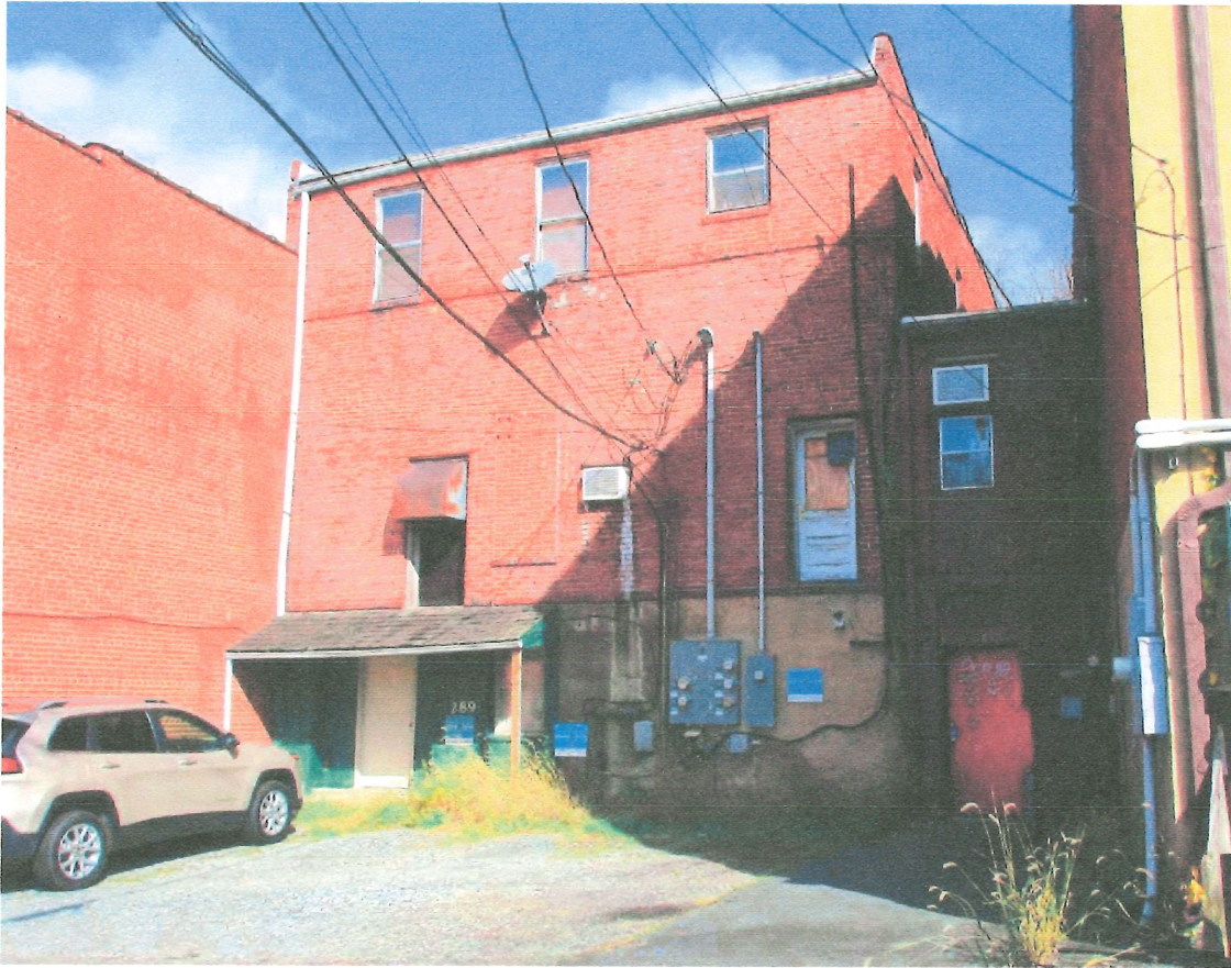
Side (east) elevation of rear of west half of Qualls Block (left) and rear (south) elevation of the east half of the Qualls Block (center) as photographed on November 12, 2015, by Nicole Holladay for the Downtown Boone Historic Resources Survey.
