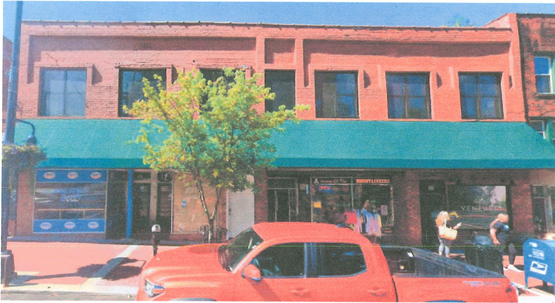
The north elevation of the Qualls Block as it appeared in August 2022, after renovation of the westernmost storefront for Venture Chocolate and replacement of the second-floor windows. Image courtesy of Google Streetview.
