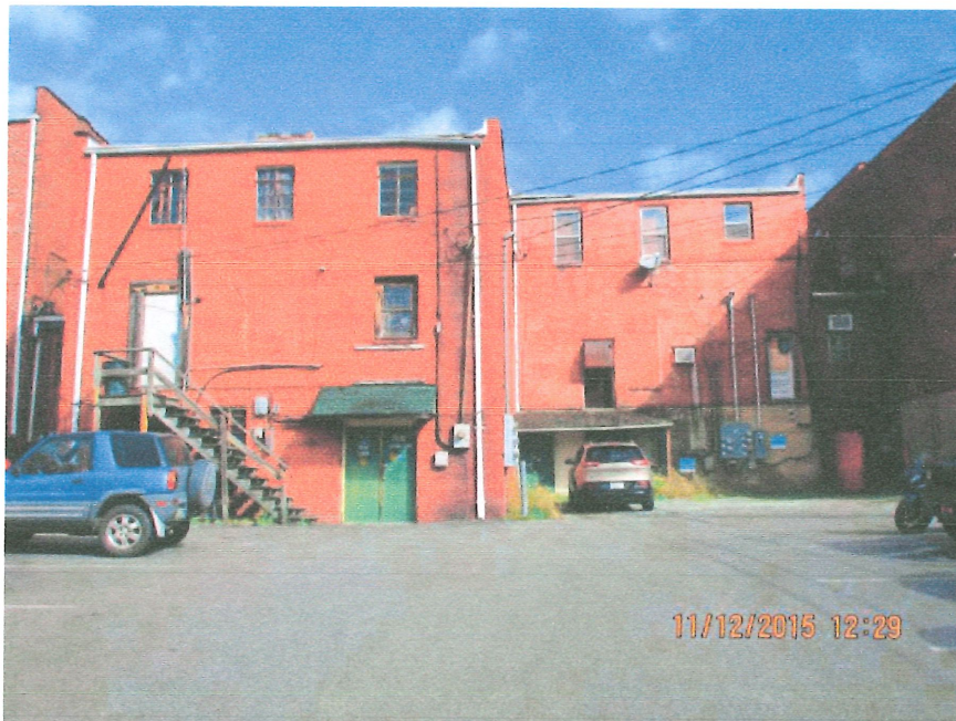
Rear (south) elevation of the Qualls Block as photographed on November 12, 2015, by Nicole Holladay for the Downtown Boone Historic Resources Survey.
