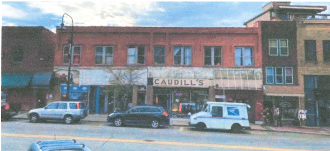
North elevation of the Qualls Block as it appeared in late 2019, after the upper façade had been painted but before the original upper façade windows had been replaced. Image provided by Will Clark, Trade Land Company LLC.
