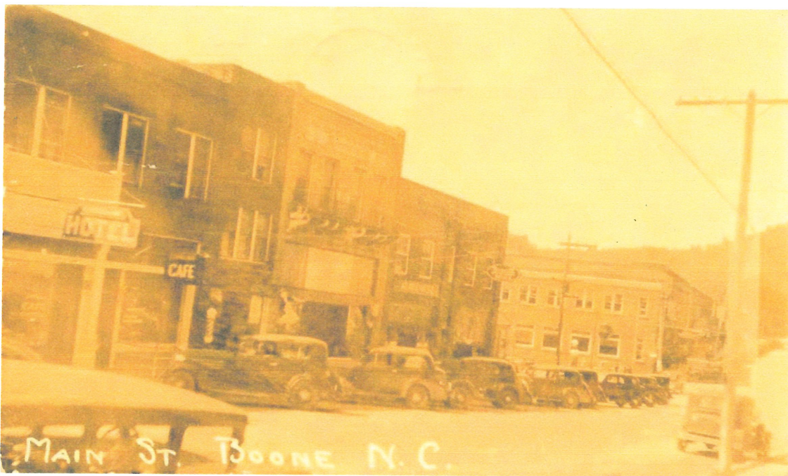
The western half of the Qualls Block (left) as it appeared with its new portico circa 1937. Image courtesy of the Bobby Brendell Postcard Collection, Digital Watauga Project.
