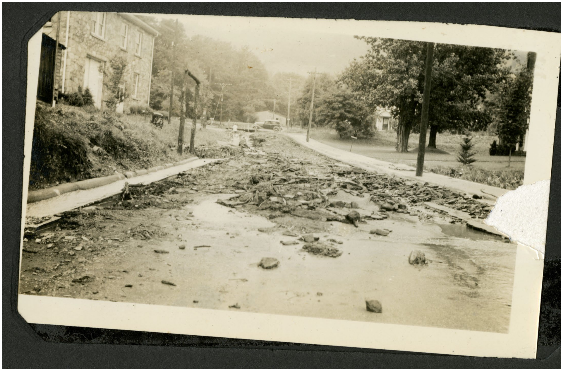
Figure 3. Paul Weston, "Flood Damage, North Water Street #2, Boone, NC, August 1940," Digital Watauga, accessed April 27, 2023, http://digitalwatauga.org/items/show/6345 .
