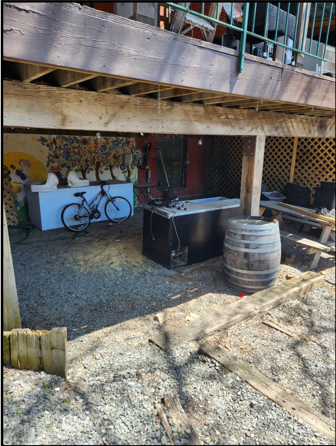
Figure 8: SEBB Under deck area – April 18, 2023.
