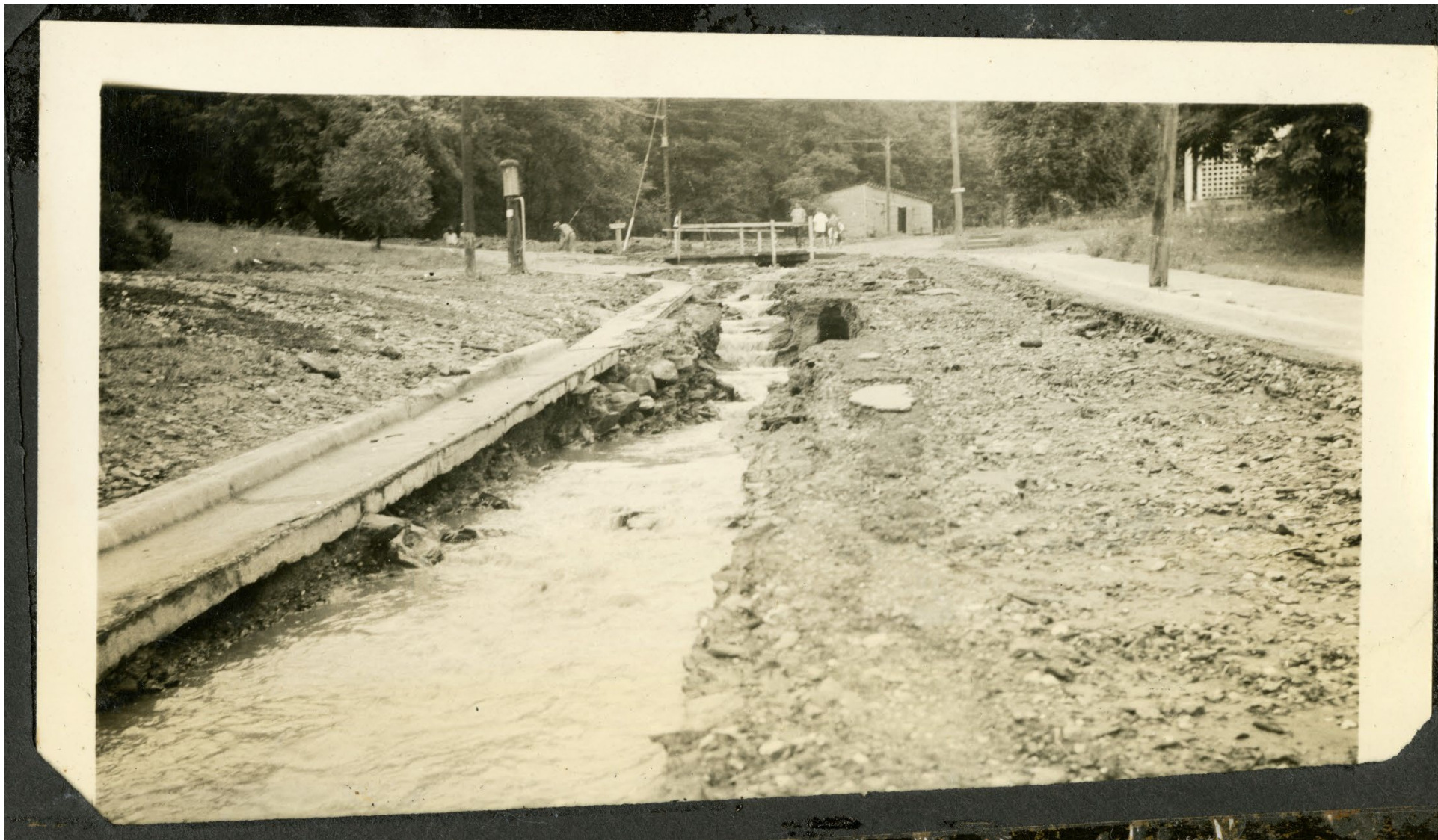
Figure 4. Paul Weston, "Flood Damage, North Water Street #3, Boone, NC, August 1940," Digital Watauga, accessed April 27, 2023, http://digitalwatauga.org/items/show/6346 .
