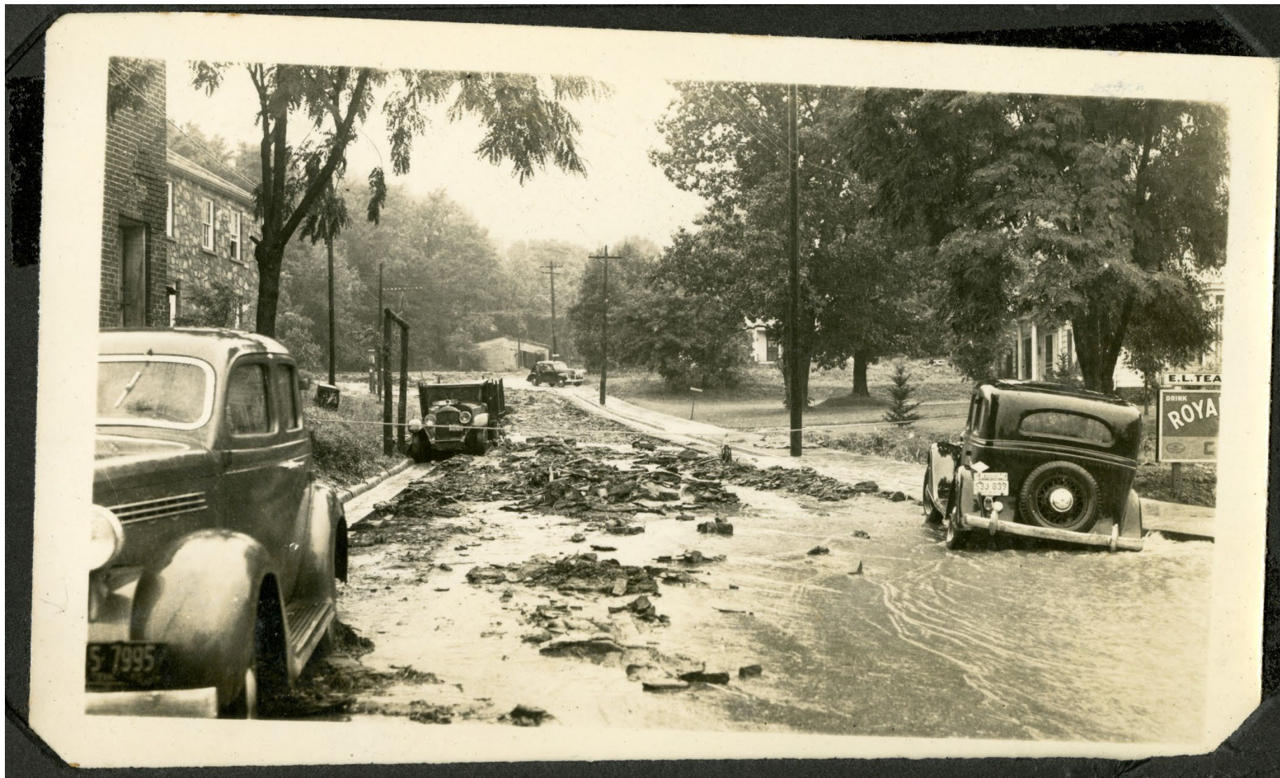
Figure 2. Paul Weston, "Flood Damage, North Water Street, Boone, NC, August 1940," Digital Watauga, accessed April 27, 2023, http://digitalwatauga.org/items/show/6344 .
