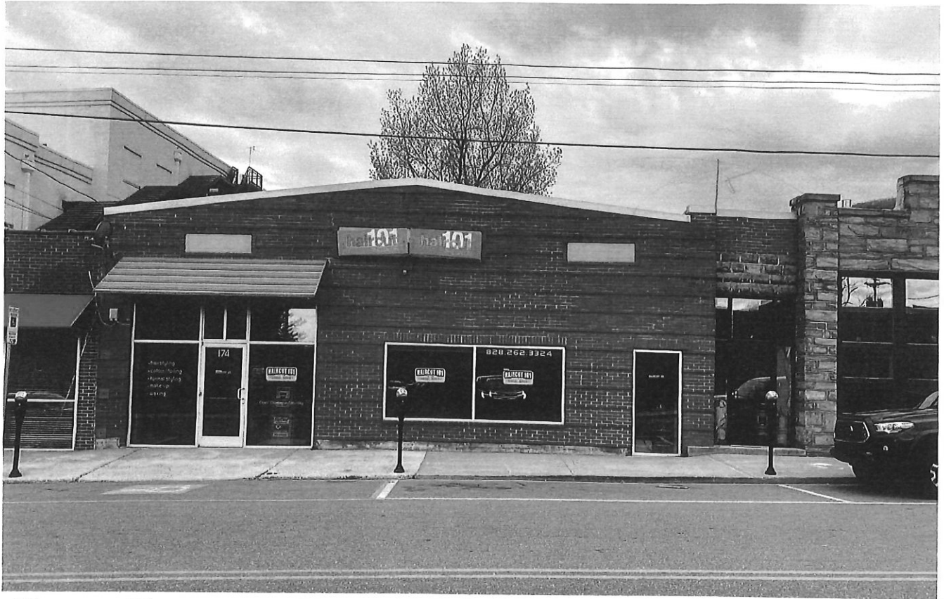
FRONT FACADE - DEPOT STREET
