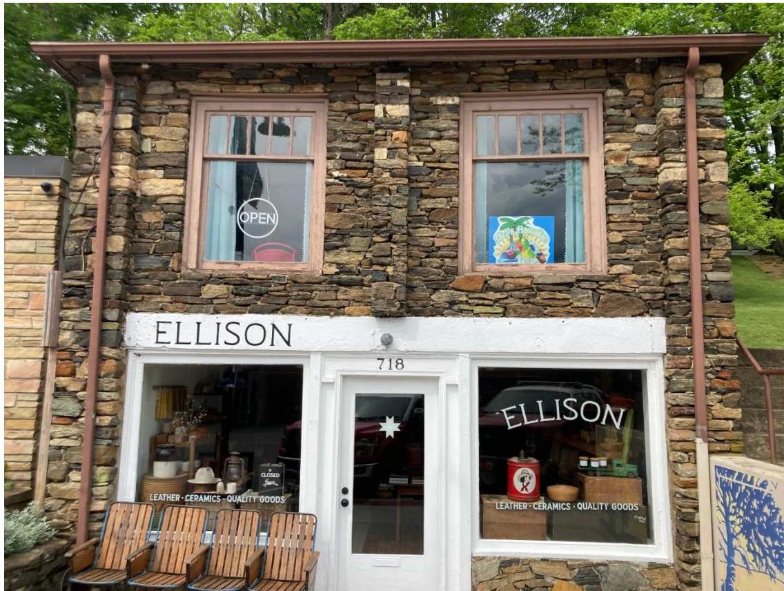
718 West King Street (WT0587). A Certificate of Appropriateness was issued on October 10, 2023, for removal of an awning, which has been completed.
