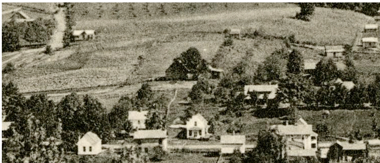
This detail crop from a circa 1915 postcard view from the south shows the area above King Street (lower foreground). At left center is the large tree visible in the 1885 and 1905 images with structures now adjacent to the tree. Lots 24 and 31 are immediately to the west and northwest (left) of the tree and still show no development. Image courtesy of the Bobby Brendell Postcard Collection, Digital Watauga Project.
