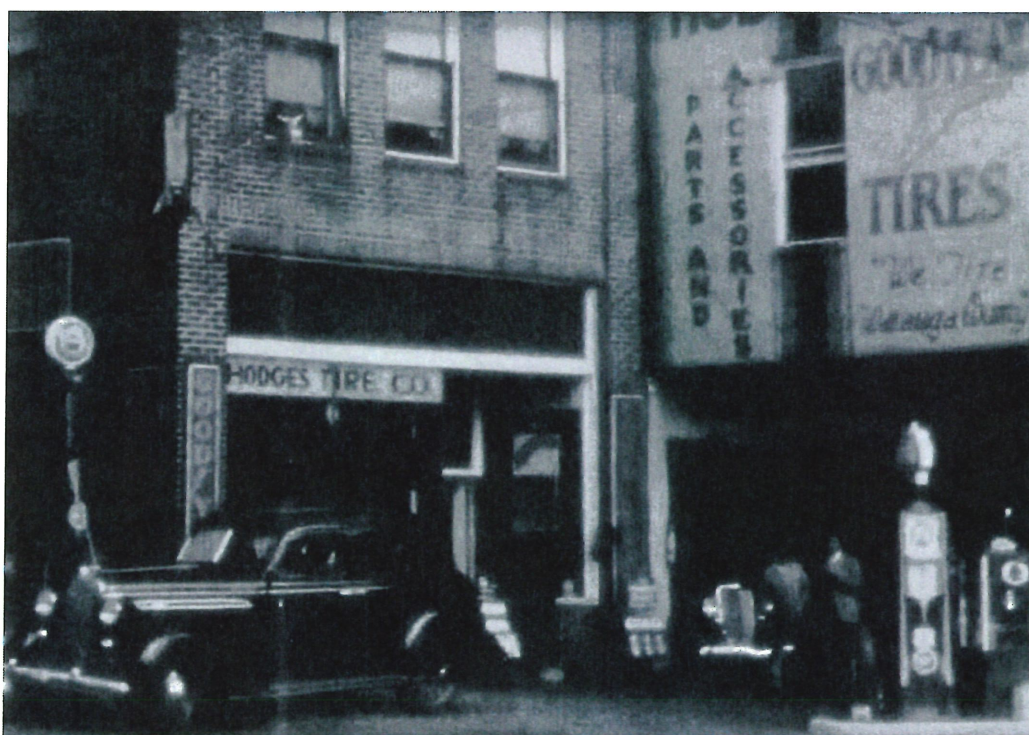
Screenshot from the 1936 H. Lee Waters film of Boone showing the west and south elevations of the W. R. Winkler Tire Company Building at left, with the west wall of the Boone Garage at right. Image courtesy of the Pilar Fotta Collection, Digital Watauga Project.
