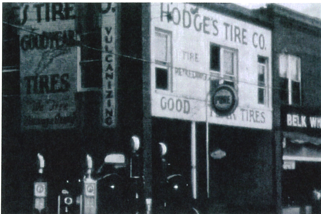
Screenshot from the 1936 H. Lee Waters film of Boone showing the Boone Garage, occupied by the Hodges Tire Company, with its south facade aligned with the south facade of the Jones Building to the east. Image courtesy of the Pilar Fotta Collection, Digital Watauga Project.
