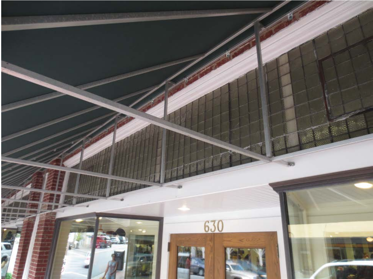
Original clerestory windows, like these found on one West King Street property, contain elaborate details that contribute to the character, appearance, and integrity of the downtown historic district. Photo courtesy of Eric Plaag, 2013.
