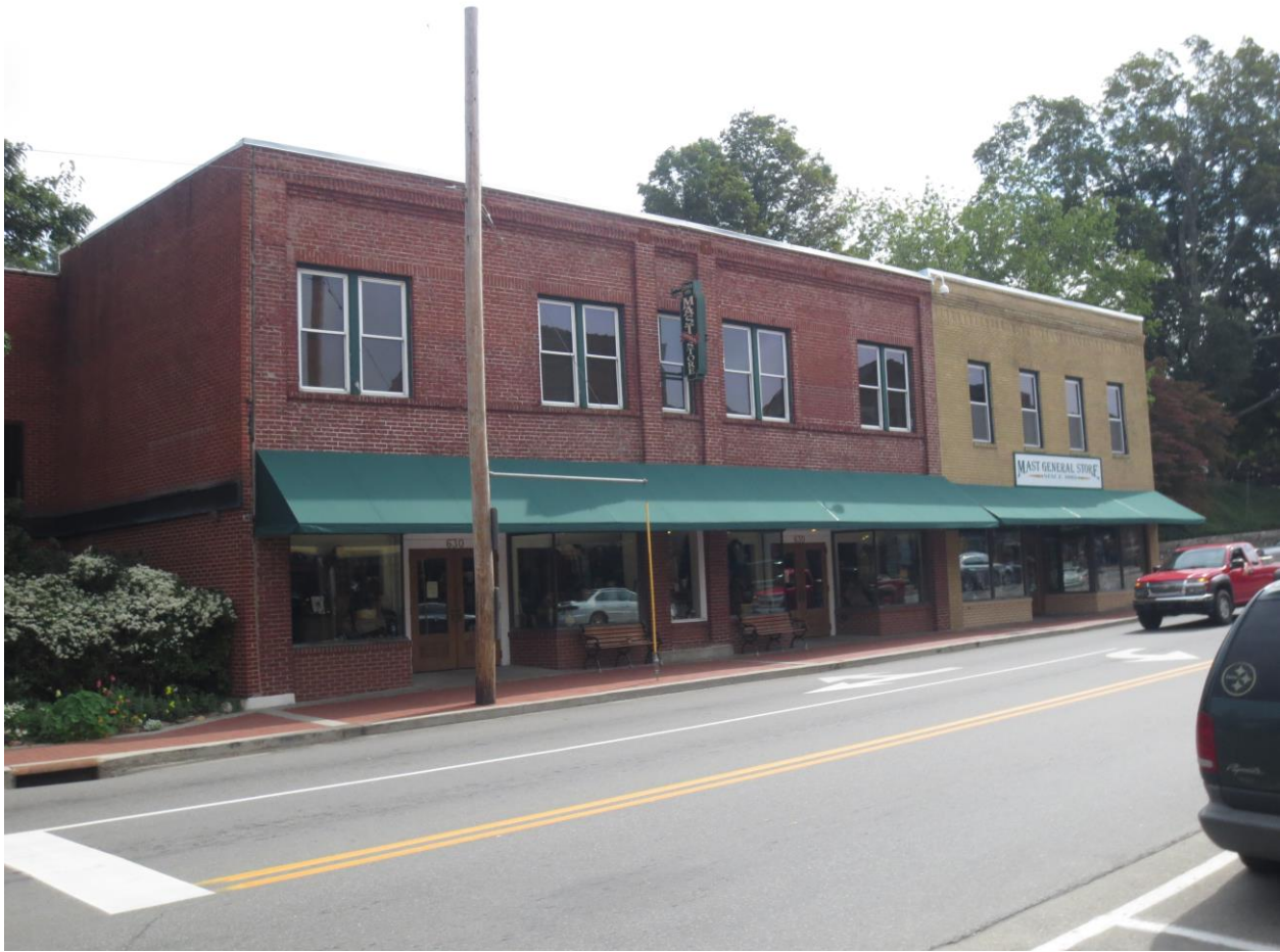
Retaining original masonry configurations, patterns, and detailing is essential to preserving the architectural character of Boone's historic districts. Photo courtesy of Eric Plaag, 2013.
