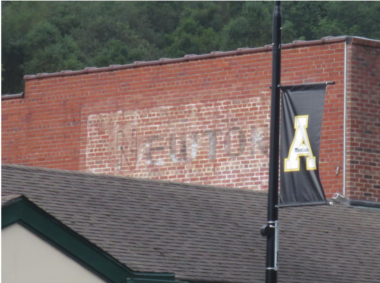
Historic “ghost ad” on the upper portion of a Downtown Boone building. Such elements are essential to the history and character of commercial historic districts and should be preserved whenever possible. Photo courtesy of Eric Plaag, 2013.
