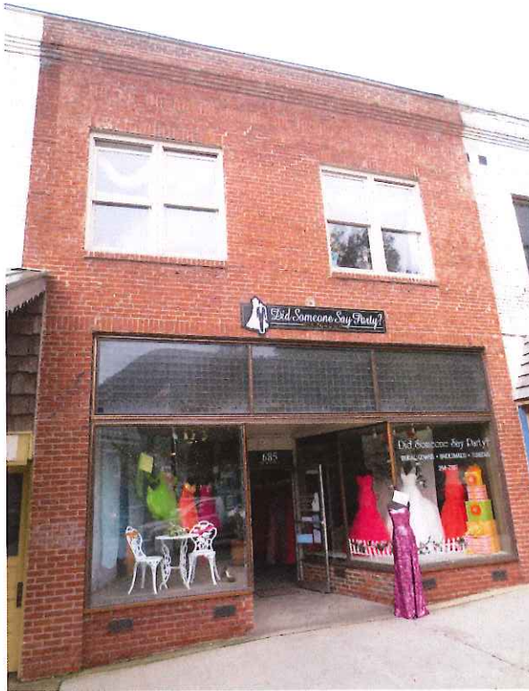
This West King Street building is an outstanding example of successful façade restoration and preservation that uncovered numerous original storefront details, including the clerestory windows above the shop windows and entrance. Photo courtesy of Eric Plaag, 2013.
