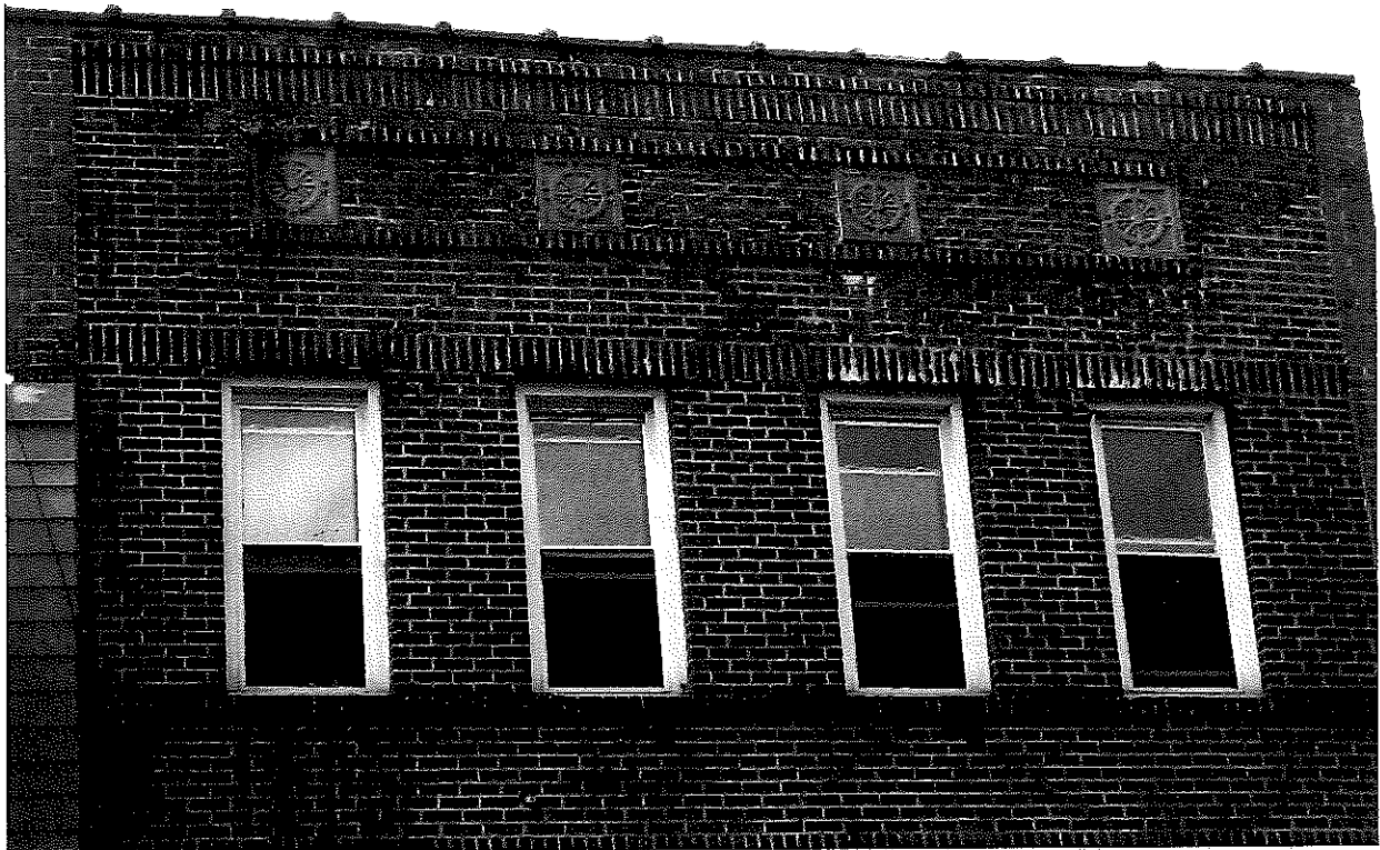
This West King Street property has suffered from poor attempts at re-pointing the masonry between the roofline and upper story windows. Photo courtesy of Eric Plaag, 2013.
