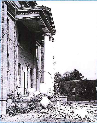
Demolition of the 1905 Watauga County Courthouse, 1967, Paul Armfield Coffey Collection, Digital Watauga Project
