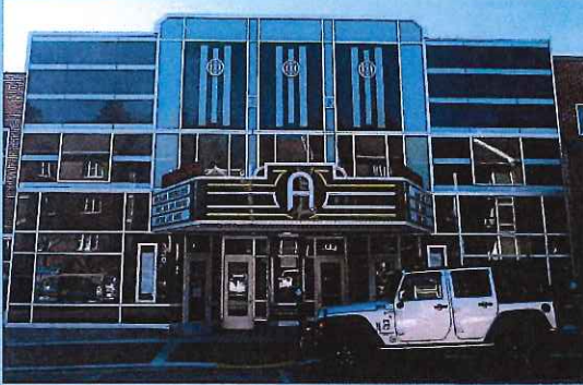
The Appalachian Theatre (1938) was completely stripped of its original facade in 2007, but the ATHC completed an historically faithful reconstruction of the facade and marquee in 2017.
