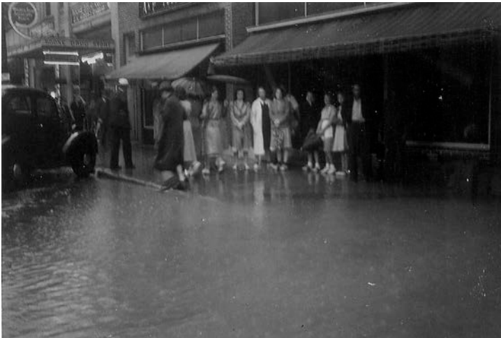
The historic Boone Drug flat awning supported by cables anchored to the façade is visible to the far left in this photo of the effects of the 1940 Boone Flood along King Street. Where possible, original awning configurations like this one should be restored to historic downtown buildings. Photo courtesy of Becky Haney-David Wyke Collection and Digital Watauga Project .
