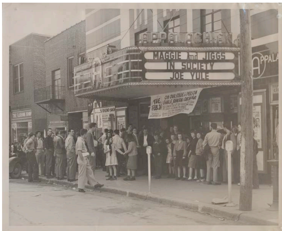
West King St., looking southeast, with Appalachian Theatre on the right, 1947. Image courtesy of The Appalachian Theatre of the High Country.
