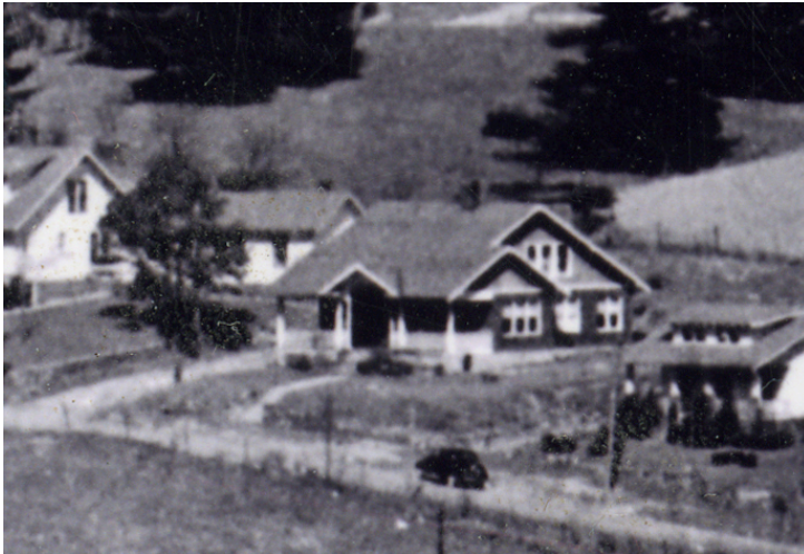
The house at 224 Grand Blvd. as it appeared in 1939. Detail from historic 1939 image of Boone, courtesy of Robert Snead and the Town of Boone Cultural Resources Department.
