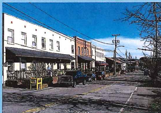
Infrastructure improvements will make Howard St. one way from Appalachian St. to Water St. and more pedestrian friendly.
