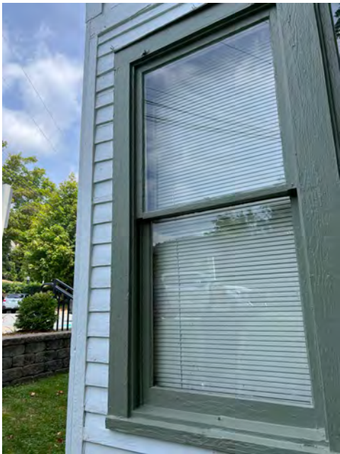
64. NC_WataugaCounty_JohnWatlerJonesHouse_0064. J PG Jones House, west elevation detail, looking northeast
