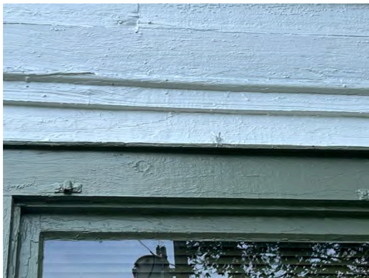
65. NC_WataugaCounty_JohnWatlerJonesHouse_0065. J PG Jones House, west elevation detail, looking east
