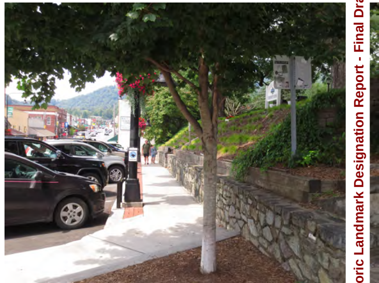
12. NC_WataugaCounty_JohnWatlerJonesHouse_001 J P G Jones House, retaining wall, looking west
