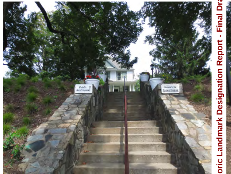
16. NC_WataugaCounty_JohnWatlerJonesHouse_001 J PG Jones House, retaining wall steps, looking north
