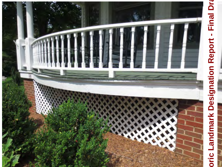
32. NC_WataugaCounty_JohnWatlerJonesHouse_0032. J PG Jones House, brick peers and white lattice, looking north
