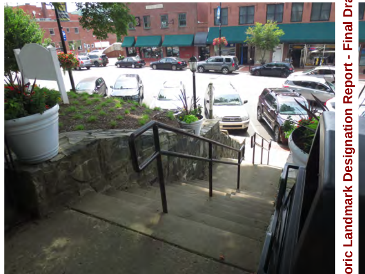
20. NC_WataugaCounty_JohnWatlerJonesHouse_002 J PG Jones House, retaining wall steps, looking southeast from Jone House lawn
