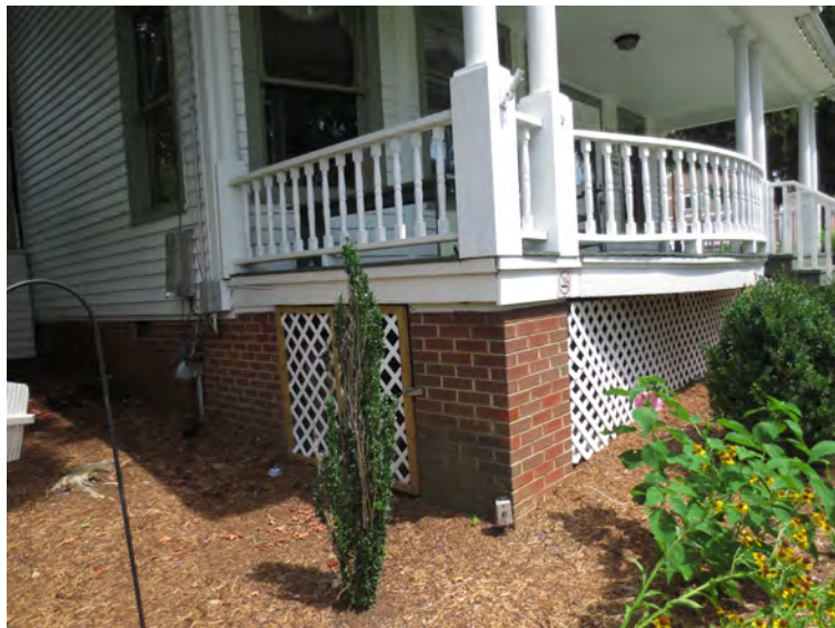
31. NC_WataugaCounty_JohnWatlerJonesHouse_0031. J PG Jones House, brick peers and white lattice, looking northeast
