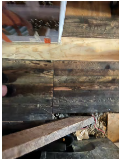
74. NC_WataugaCounty_JohnWatlerJonesHouse_007 J PG Jones House, interior attic flooring
