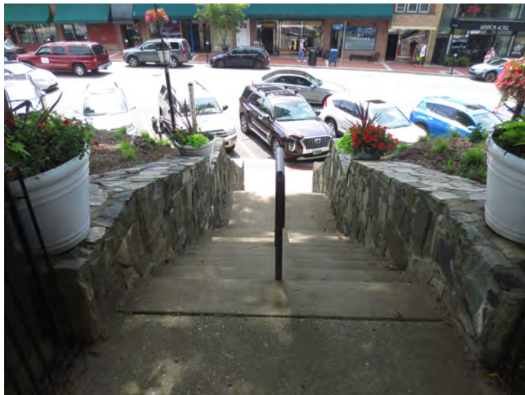
19. NC_WataugaCounty_JohnWatlerJonesHouse_0019. J PG Jones House, retaining wall steps, looking south from Jones House lawn
