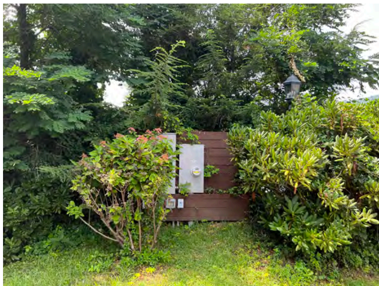
57. NC_WataugaCounty_JohnWatlerJonesHouse_0057. J PG Jones House, electric box on lawn
