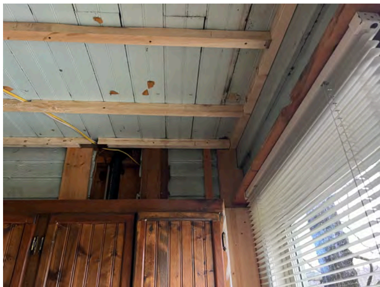
119. NC_WataugaCounty_JohnWatlerJonesHouse_0119.J P G Jones House, interior detail
