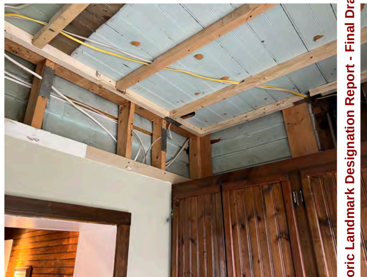
120. NC_WataugaCounty_JohnWatlerJonesHouse_0120.J P G Jones House, interior detail
