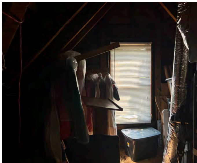
76. NC_WataugaCounty_JohnWatlerJonesHouse_007 PG Jones House, interior attic detail, looking south
