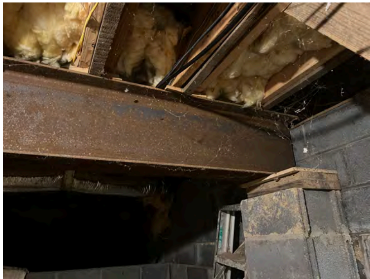
71. NC_WataugaCounty_JohnWatlerJonesHouse_0071.J P G Jones House, interior basement detail,
