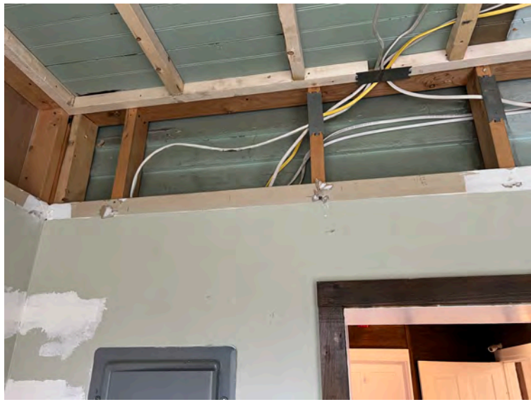
121. NC_WataugaCounty_JohnWatlerJonesHouse_0121.J P G Jones House, interior detail
