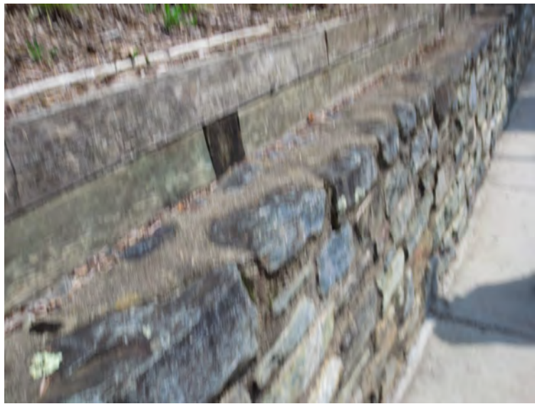
9. NC_WataugaCounty_JohnWatlerJonesHouse_0009. J P G Jones House, retaining wall, looking east
