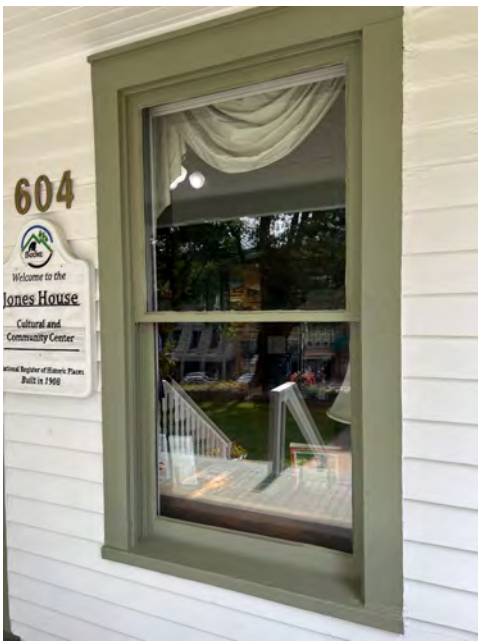
45. NC_WataugaCounty_JohnWatlerJonesHouse_0045. J PG Jones House, south entrance detail
