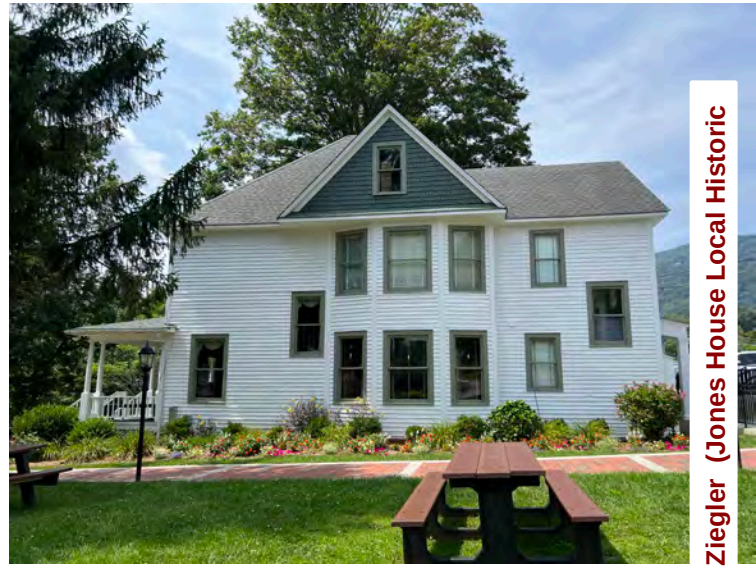
46. NC_WataugaCounty_JohnWatlerJonesHouse_004 J PG Jones House, east elevation, looking west
