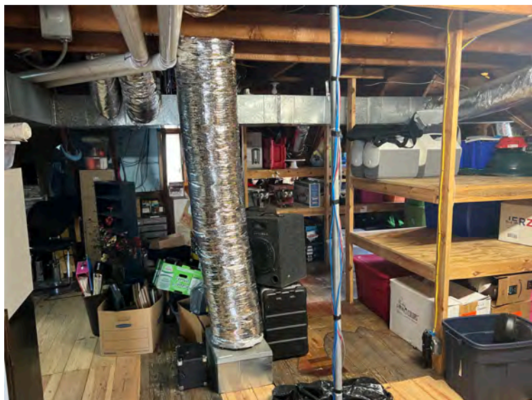
75. NC_WataugaCounty_JohnWatlerJonesHouse_0075. J PG Jones House, interior attic, looking east
