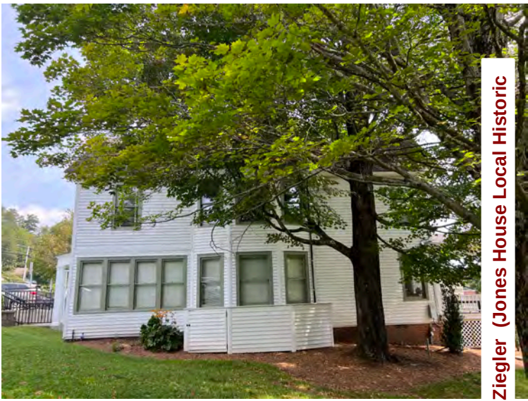
62. NC_WataugaCounty_JohnWatlerJonesHouse_0062. J PG Jones House, west elevation and landscape, looking east
