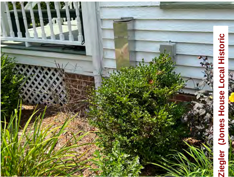
50. NC_WataugaCounty_JohnWatlerJonesHouse_0050. J PG Jones House, east elevation detail, looking west
