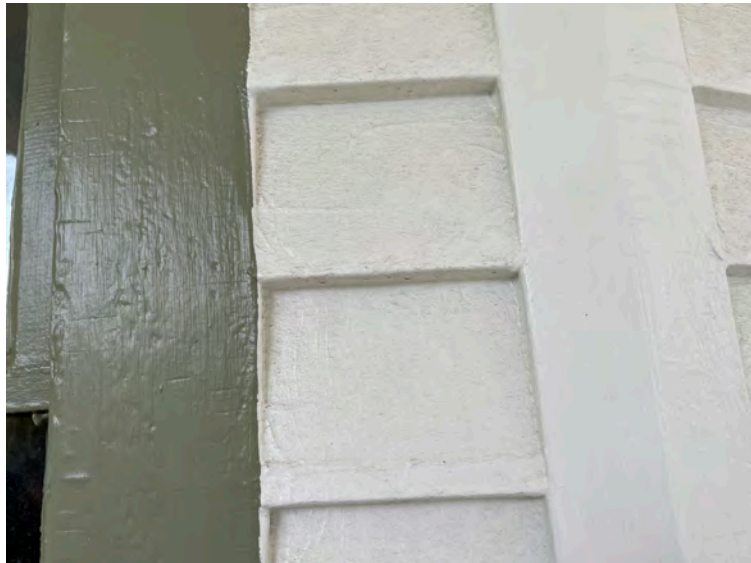
39. NC_WataugaCounty_JohnWatlerJonesHouse_0039. J P G Jones House, southern facade detail
