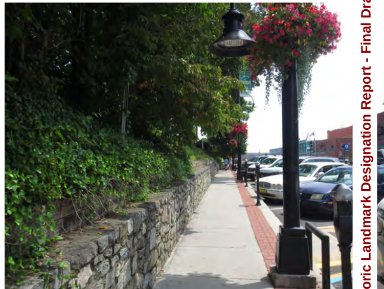
8. NC_WataugaCounty_JohnWatlerJonesHouse_0008. J P G The Jones House retaining wall, looking east from King Street
