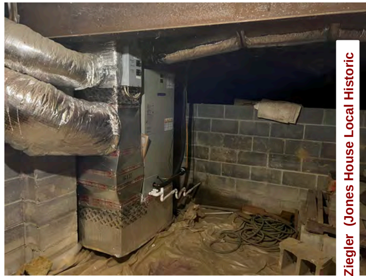
70. NC_WataugaCounty_JohnWatlerJonesHouse_0070. J PG Jones House, interior basement, looking southwest
