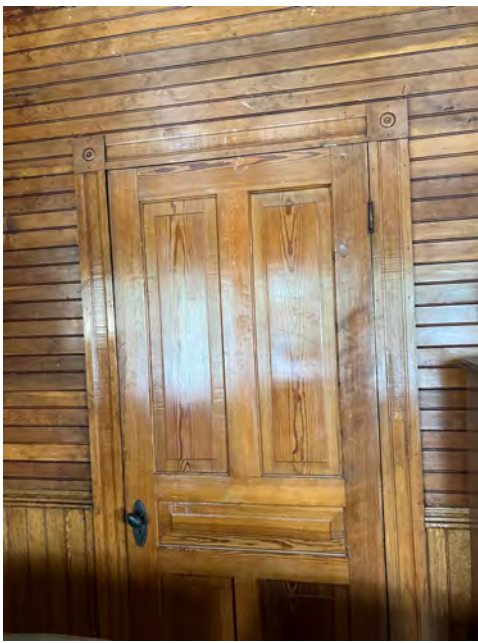
113. NC_WataugaCounty_JohnWatlerJonesHouse_0113.J P G Jones House, interior detail
