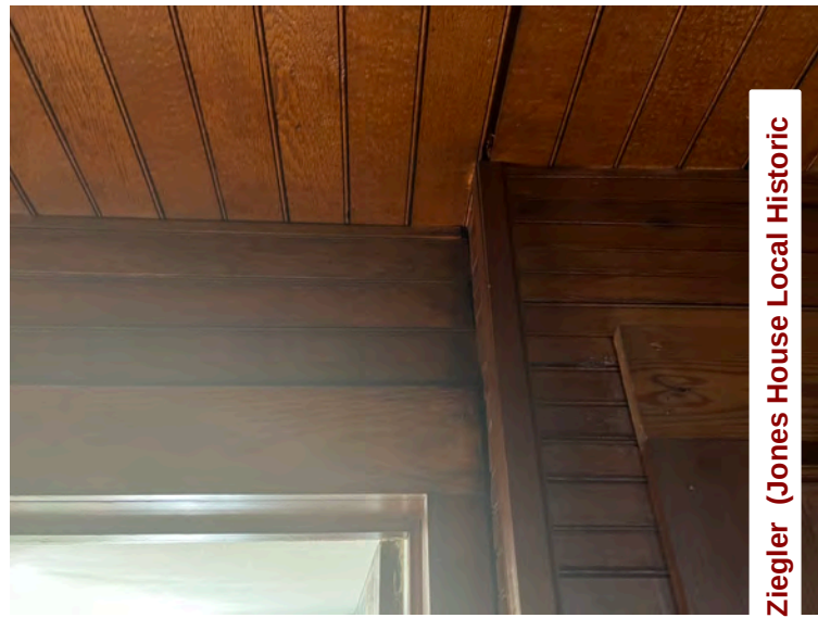
98. NC_WataugaCounty_JohnWatlerJonesHouse_0098. J P G Jones House, interior detail, looking south
