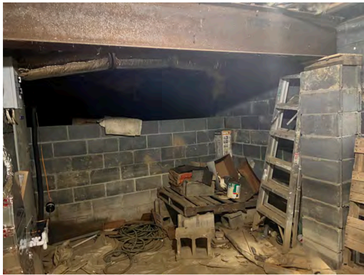
69. NC_WataugaCounty_JohnWatlerJonesHouse_0069. J PG Jones House, interior basement, looking southwest
