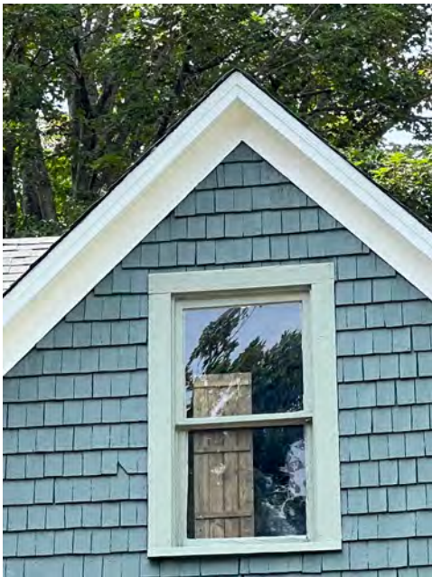
47. NC_WataugaCounty_JohnWatlerJonesHouse_0047. J PG Jones House, east elevation detail, looking west
