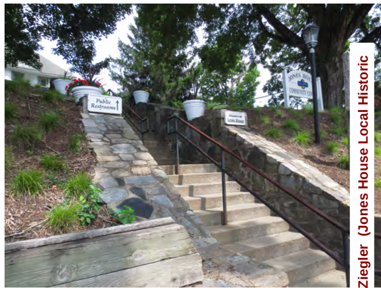
18. NC_WataugaCounty_JohnWatlerJonesHouse_001 J PG Jones House, retaining wall steps, looking northeast
