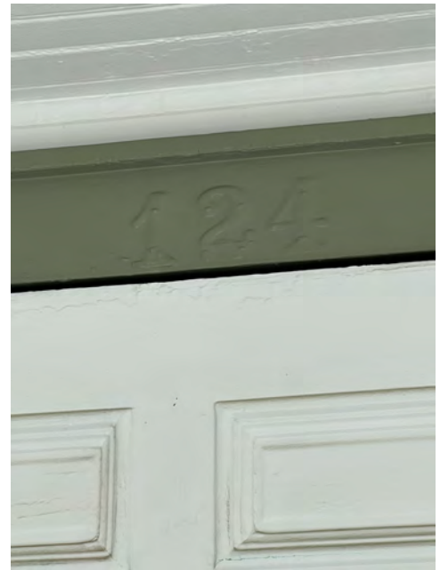
44. NC_WataugaCounty_JohnWatlerJonesHouse_0044. J PG Jones House, southern entrance detail
