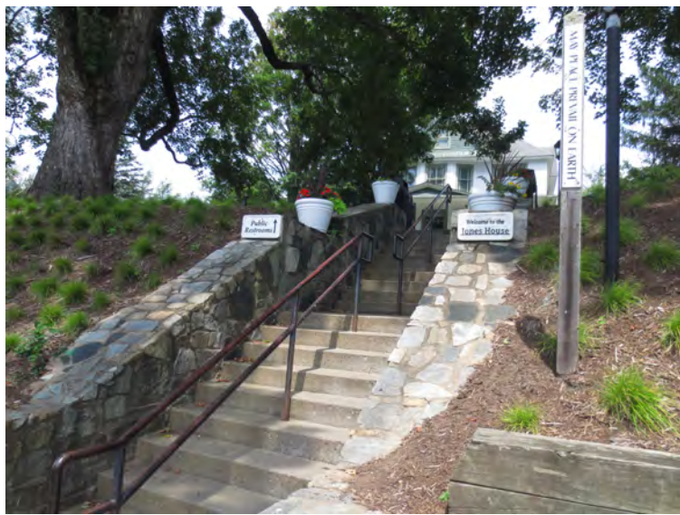
17. NC_WataugaCounty_JohnWatlerJonesHouse_0017.J P G Jones House, retaining wall steps, looking northwest
