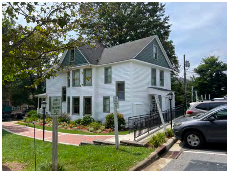
59. NC_WataugaCounty_JohnWatlerJonesHouse_0059. J PG Jones House, east and north elevations, looking west
