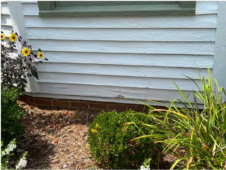
51. NC_WataugaCounty_JohnWatlerJonesHouse_0051. J PG Jones House, east elevation detail, looking west
