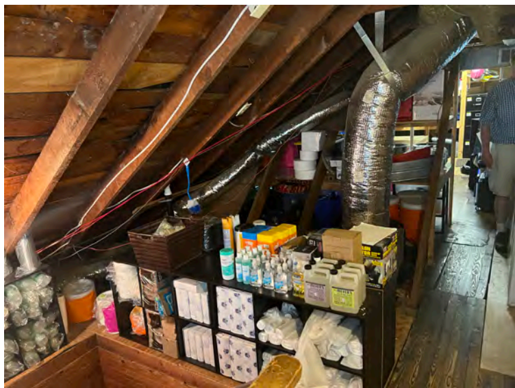
73. NC_WataugaCounty_JohnWatlerJonesHouse_0073. J PG Jones House, interior attic, looking south
