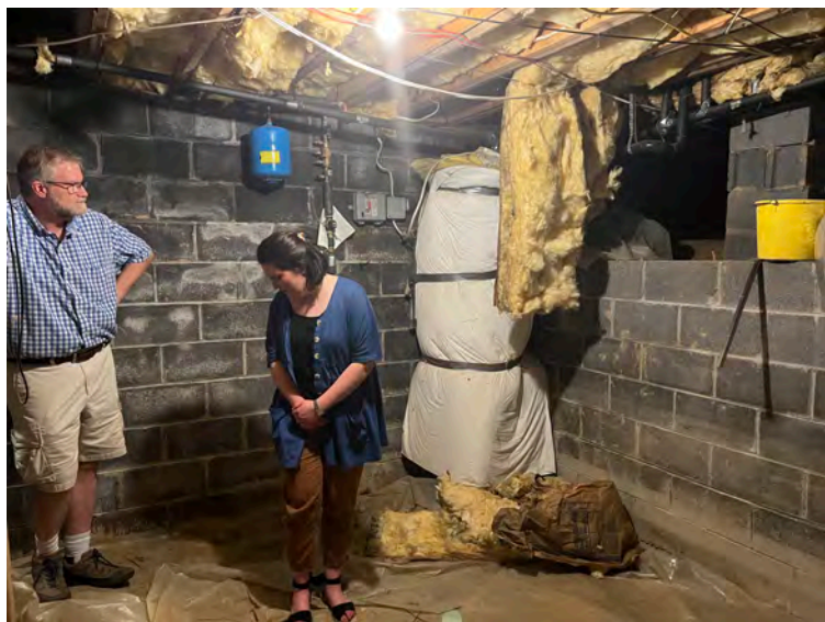
67. NC_WataugaCounty_JohnWatlerJonesHouse_0067. J PG Jones House, interior basement, looking east
