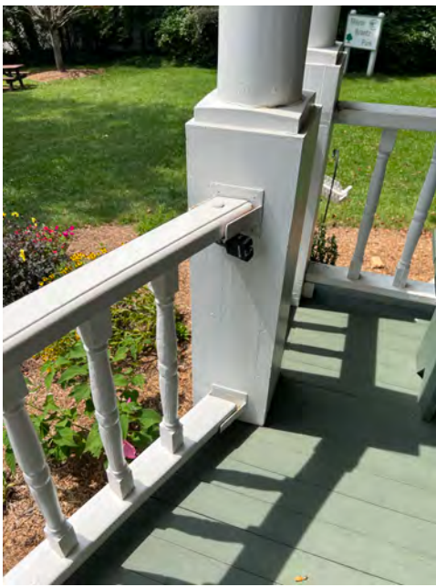
41. NC_WataugaCounty_JohnWatlerJonesHouse_0041. J PG Jones House, southern porch detail, looking southwest
