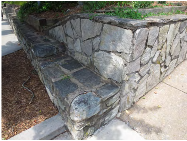
13. NC_WataugaCounty_JohnWatlerJonesHouse_0013. J PG Jones House, retaining wall, looking west
