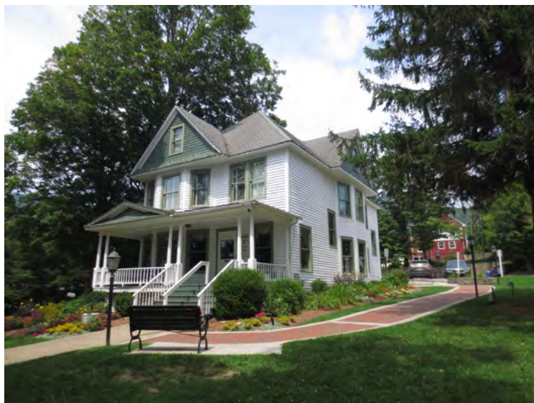
29. NC_WataugaCounty_JohnWatlerJonesHouse_0029. J PG Jones House, south and east elevations, looking northwest
