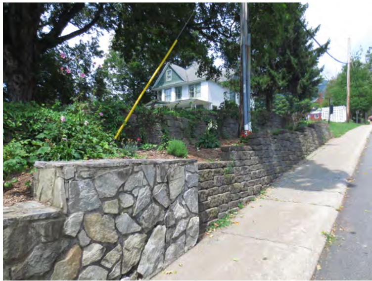
15. NC_WataugaCounty_JohnWatlerJonesHouse_0015. J PG Jones House, south elevation and retaining wall, looking Northwest
