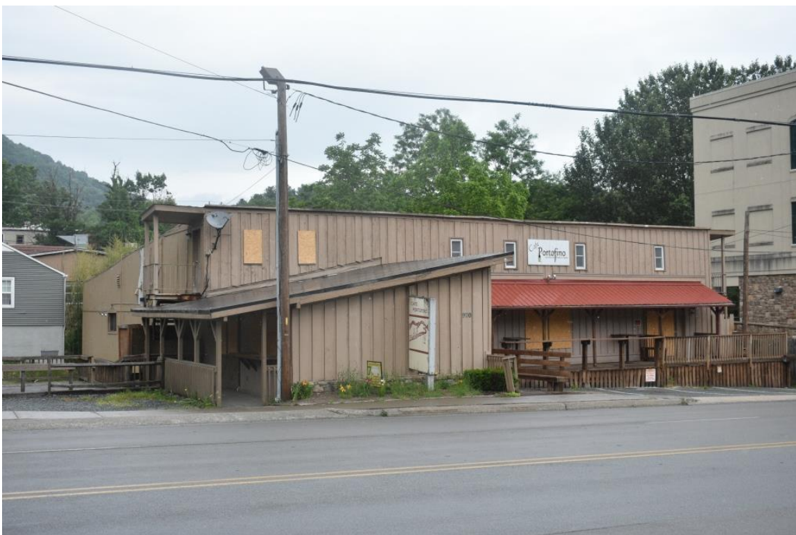
Façade, oblique view to northeast
