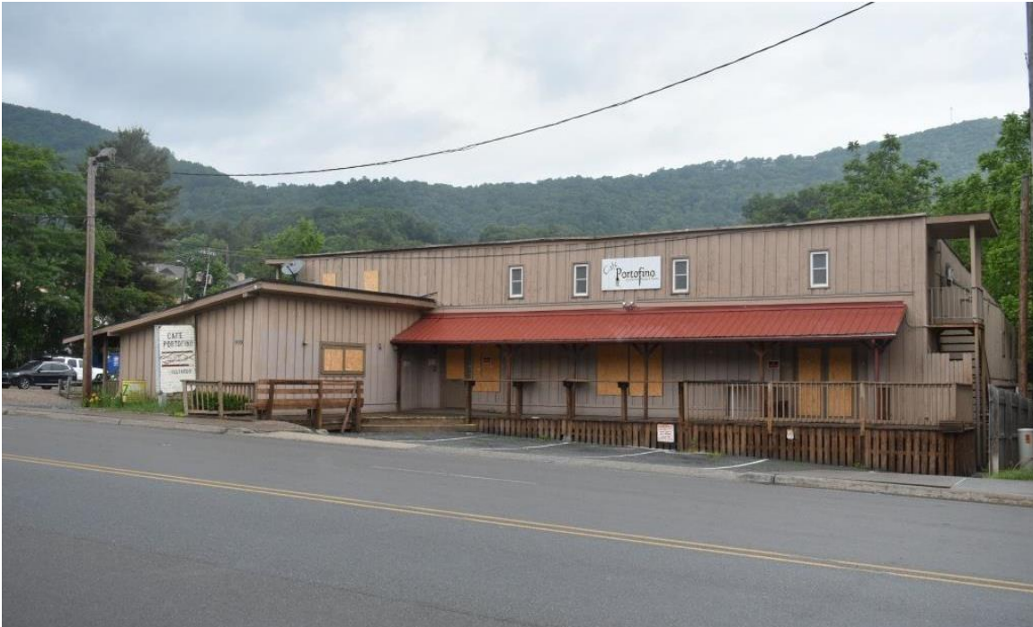
Façade, view to north
