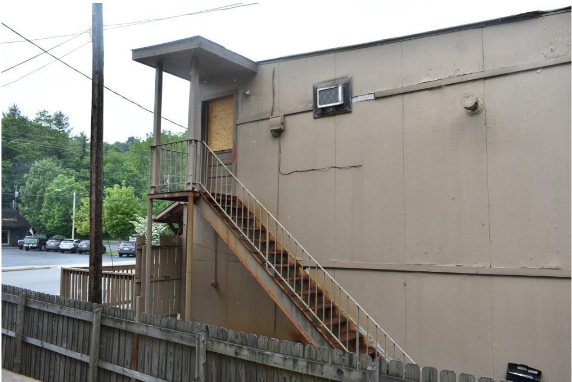
Entrance to Apt. B on southwest side elevation, view to west
