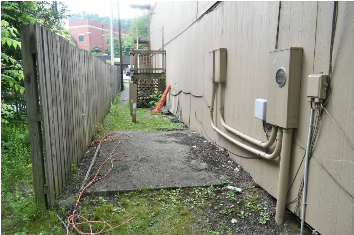
Southeast side elevation and property boundary, view to southwest
