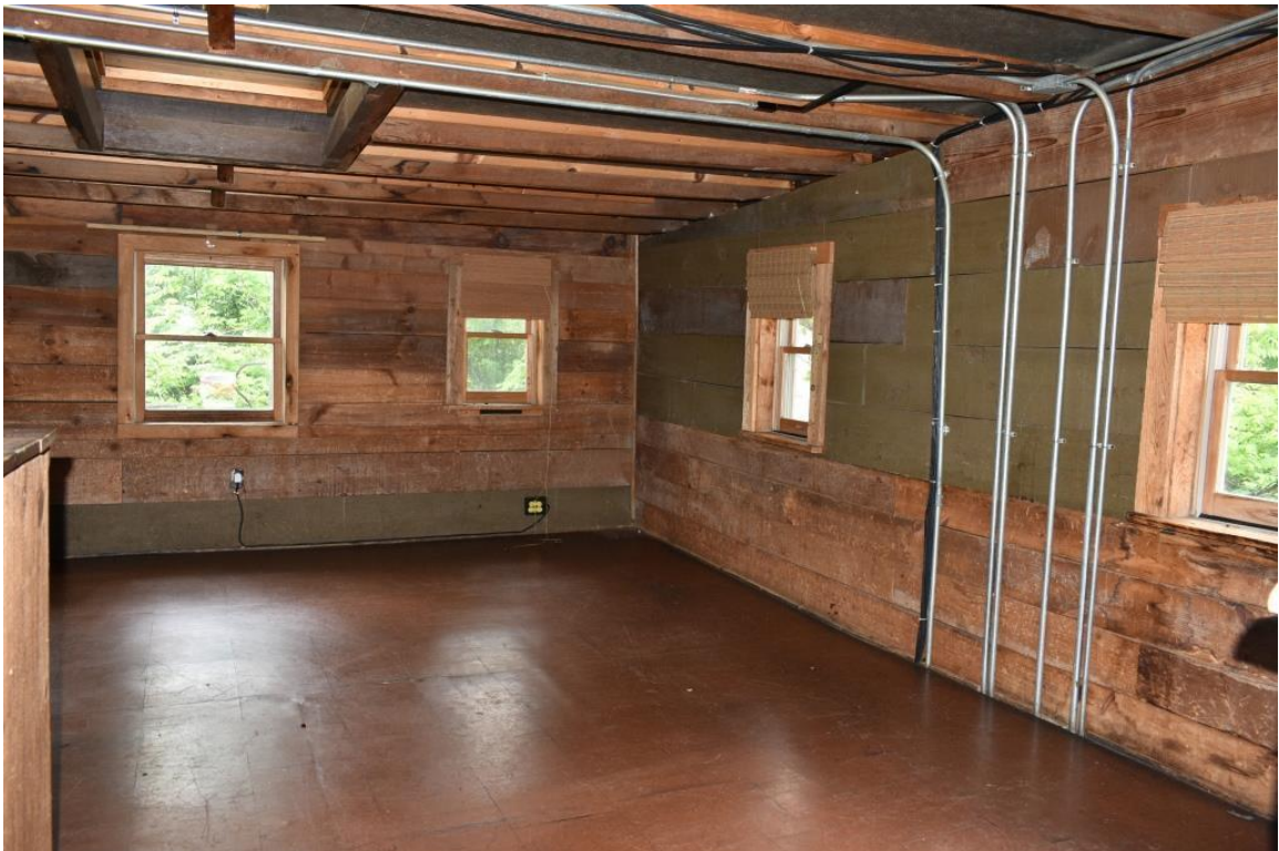
Mezzanine at northeast corner, view to northeast
