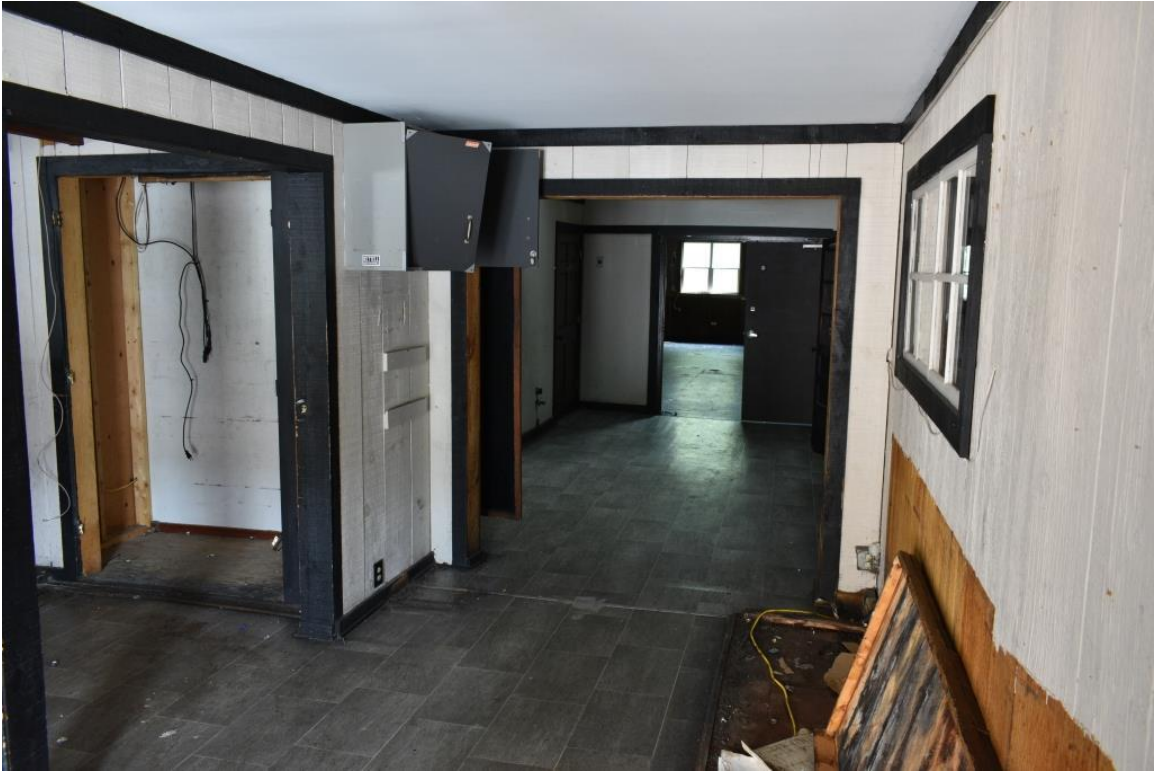
Entrance corridor for bar, view to north
