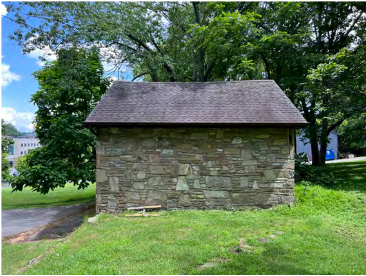
NC_WataugaCounty_RLClayHouse_0031.JPG R. L. Clay House Garage, looking southeast
