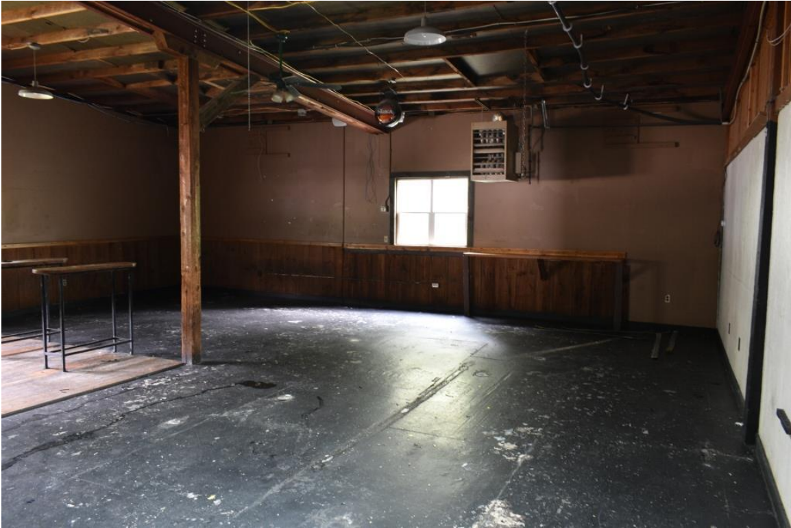
Lounge interior, view to north
