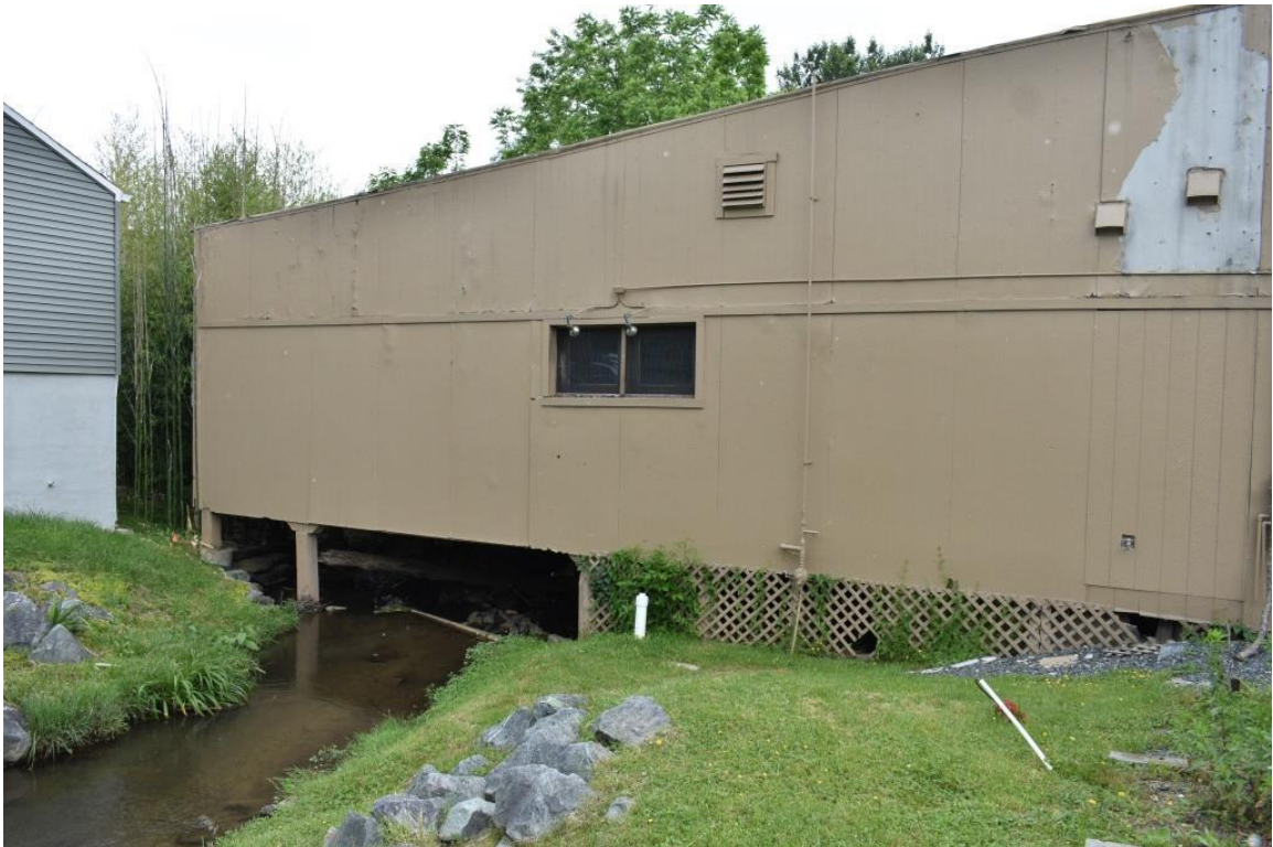
Northwest side elevation with Boone Creek below the northwest corner, view to east
