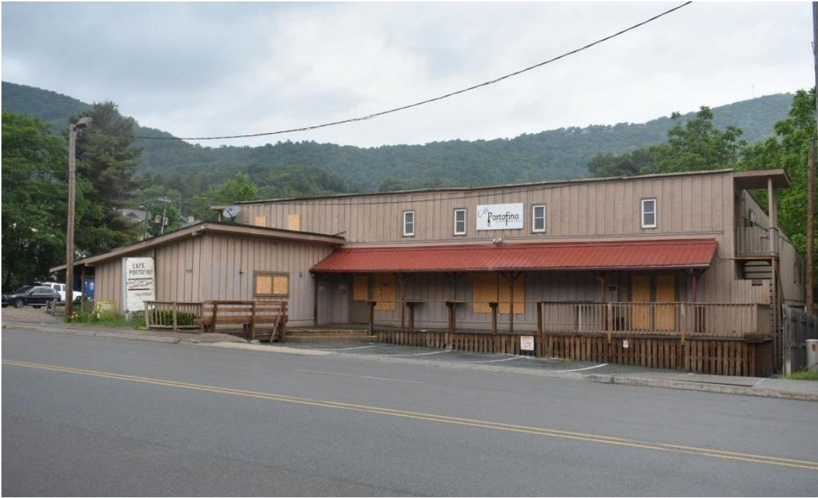
Façade, view to north
