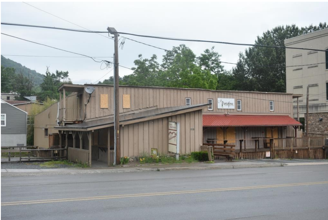
Façade, oblique view to northeast
