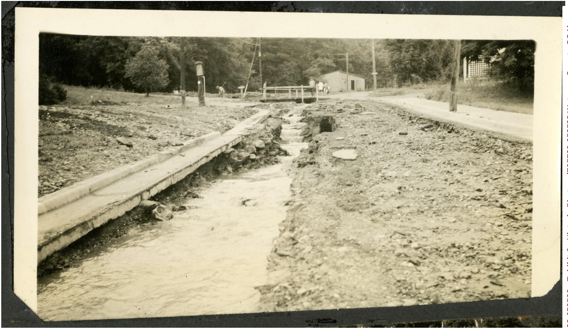
Figure 4. Paul Weston, "Flood Damage, North Water Street #3, Boone, NC, August 1940," Digital Watauga, accessed June 28, 2022, http://digitalwatauga.org/items/show/6346 .
