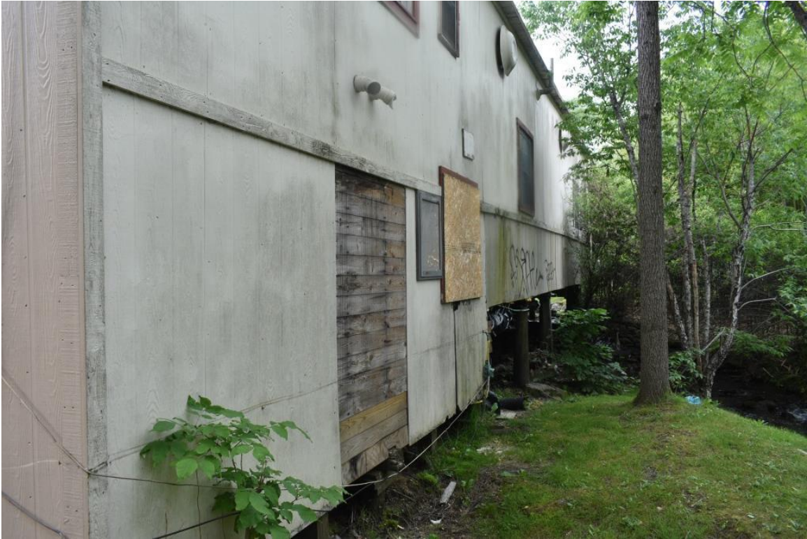
Rear elevation, oblique view to west
