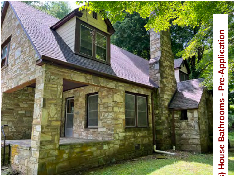
NC_WataugaCounty_RLClayHouse_0006.JPG R. L. Clay House, looking west
