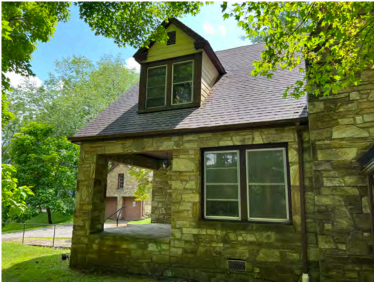
NC_WataugaCounty_RLClayHouse_0007.JPG R. L. Clay House and Garage, looking south
