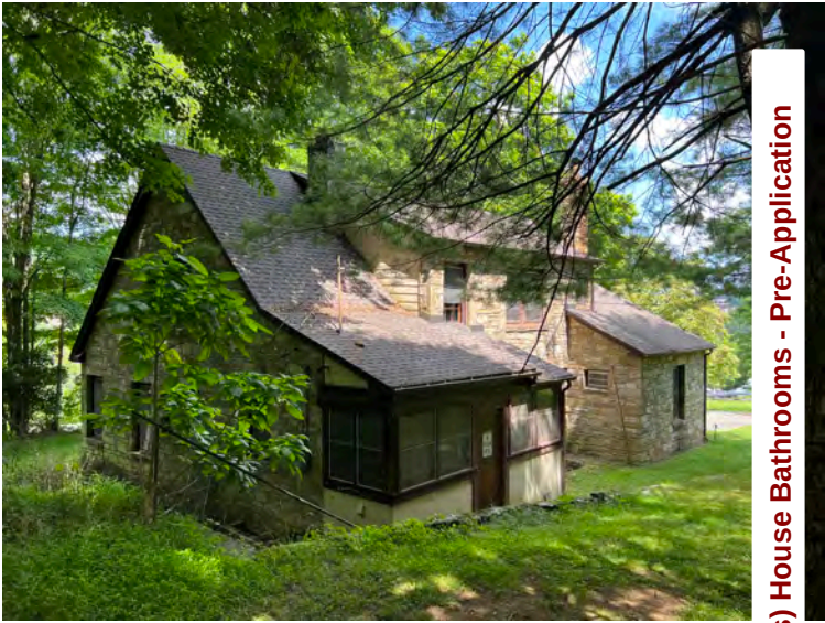
NC_WataugaCounty_RLClayHouse_0014.JPG R. L. Clay House, looking east
