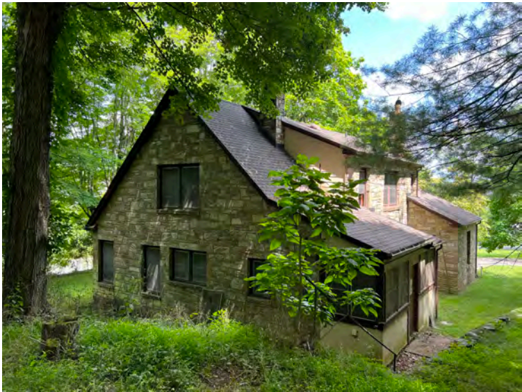
NC_WataugaCounty_RLClayHouse_0015.JPG R. L. Clay House, looking east
