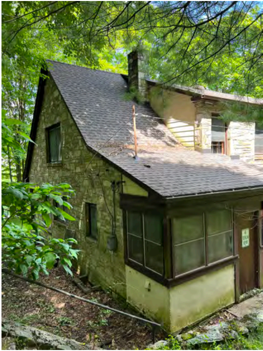
NC_WataugaCounty_RLClayHouse_0016.JPG R. L. Clay House, looking east
