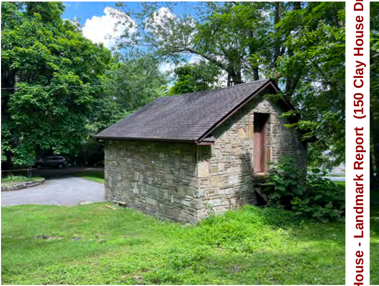
NC_WataugaCounty_RLClayHouse_0032.JPG R. L. Clay House Garage, looking east
