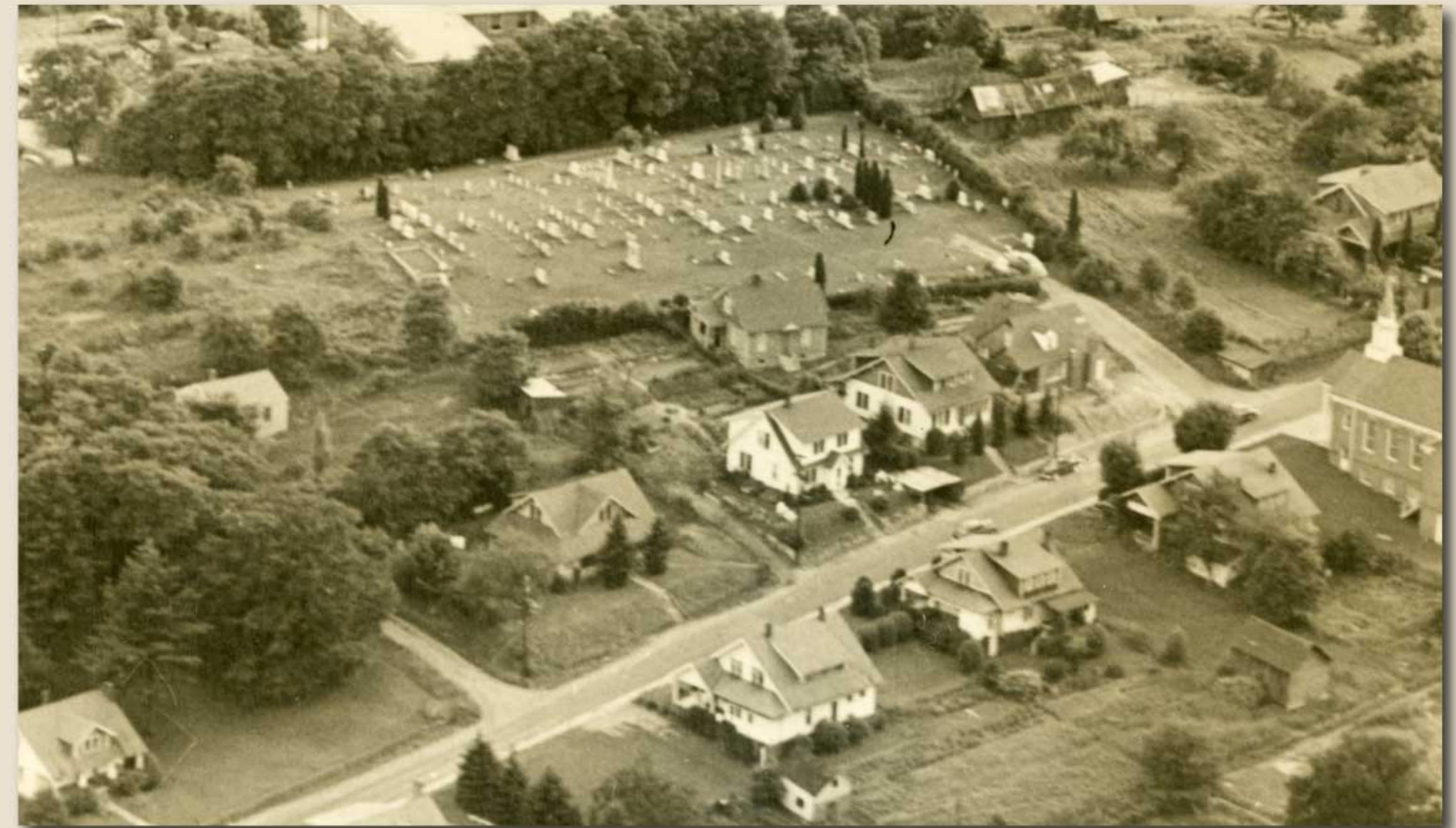
Aerial image of Boone Cemetery from the northeast, circa 1950. Image courtesy of the Blair Collection, Collection, Digital Watauga Project.
