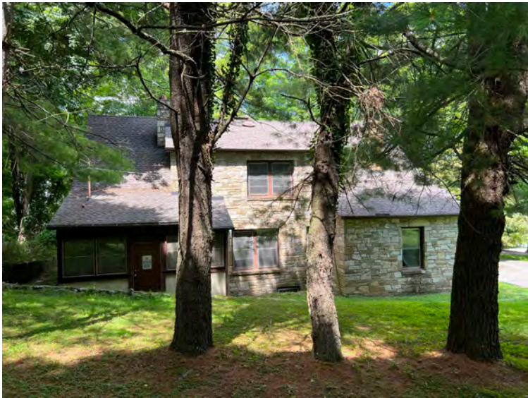
NC_WataugaCounty_RLClayHouse_0019.JPG R. L. Clay House, looking northeast
