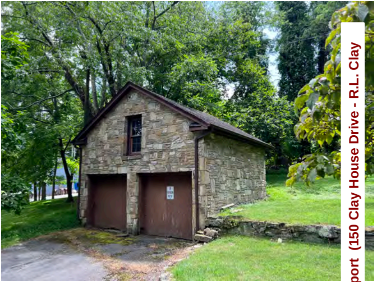
NC_WataugaCounty_RLClayHouse_0030.JPG R. L. Clay House Garage, looking south
