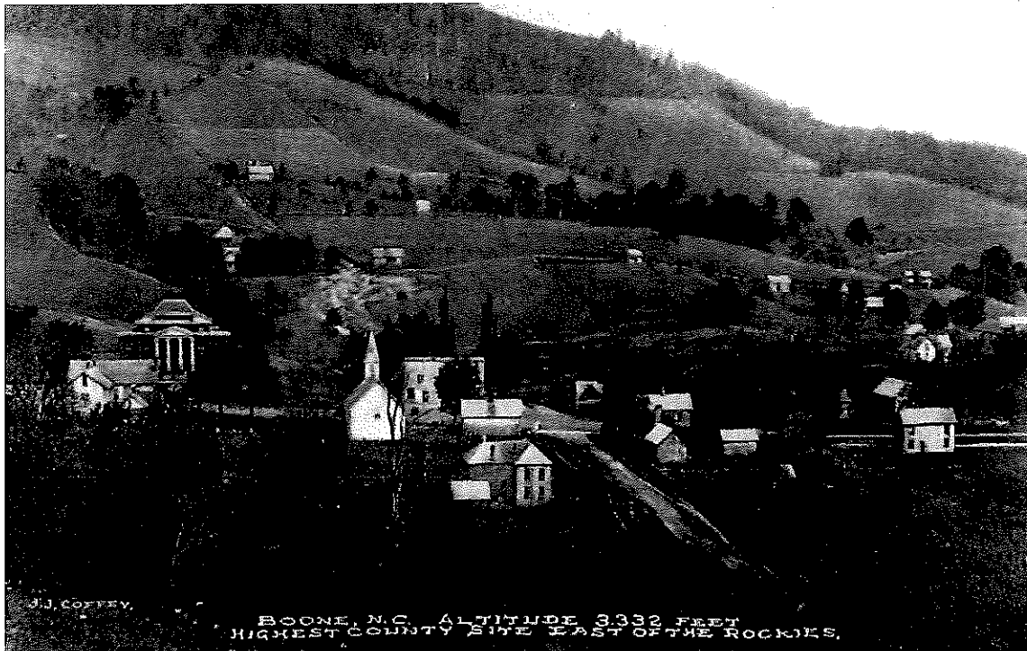
Downtown Boone from the south, as it appeared in 1905. The intersection of Water and King Streets is at center. Image courtesy of the Bobby Brendell Postcard Collection, Digital Watauga Project.
