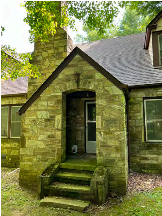
NC_WataugaCounty_RLClayHouse_0008.JPG R. L. Clay House entrance detail, looking southwest
