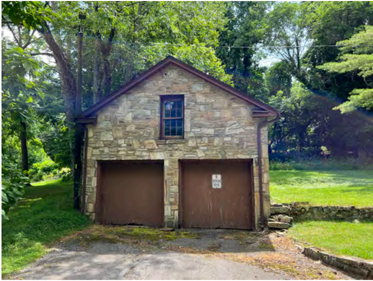
NC_WataugaCounty_RLClayHouse_0029.JPG R. L. Clay House Garage, looking southwest
