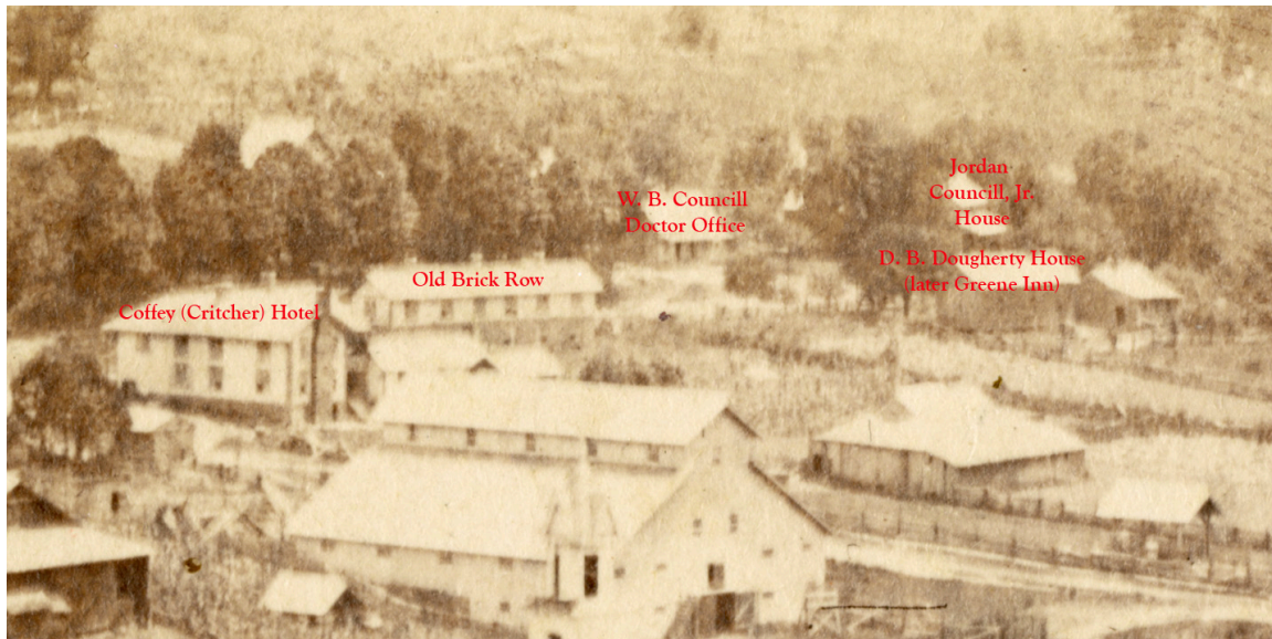
Detail crop from L. A. Ramsour's circa 1885 image of Boone from the southwest. King Street runs west to east from left to right between the Councill properties north of the road and the Old Brick Row and Dougherty House to the south of the road. Labels are speculative based on available evidence. Image from the Historic Boone Collection, Digital Watauga Project.
