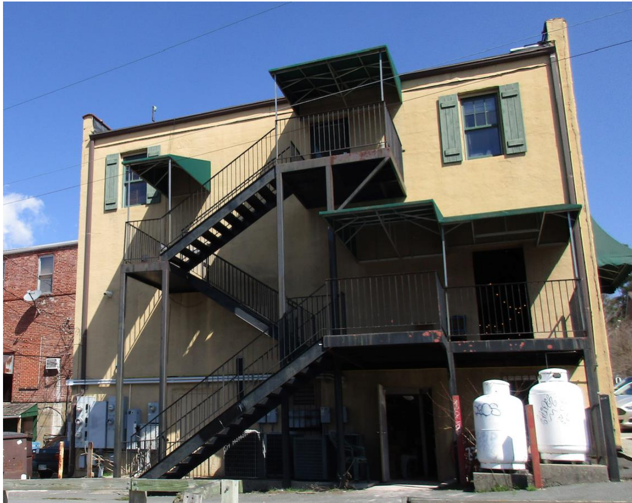
Updated fire escapes, like this one on a King Street building, should be located on a tertiary elevation not visible from streets adjacent to the primary and secondary elevations. Photo by Eric Plaag, 2016.
