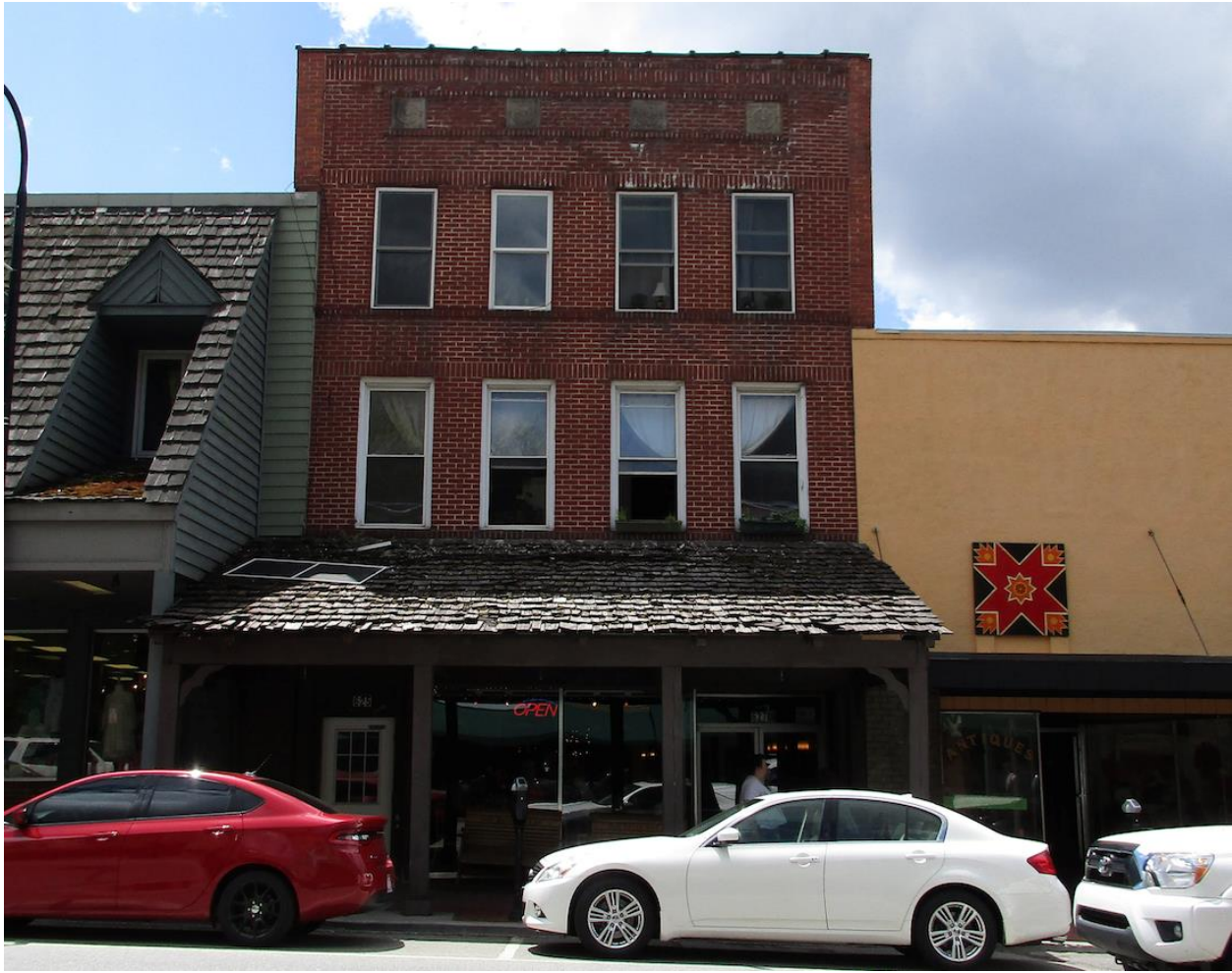
“Mountain village” porch coverings like this one on King Street are never historically appropriate to the District and should be removed in favor of historically documented metal-frame or cable-hung awnings as part of facade rehabilitation efforts. Hidden historic architectural elements, such as clerestory windows and transoms, should also be uncovered and restored. Photo by Paul Fuller, 2016.
