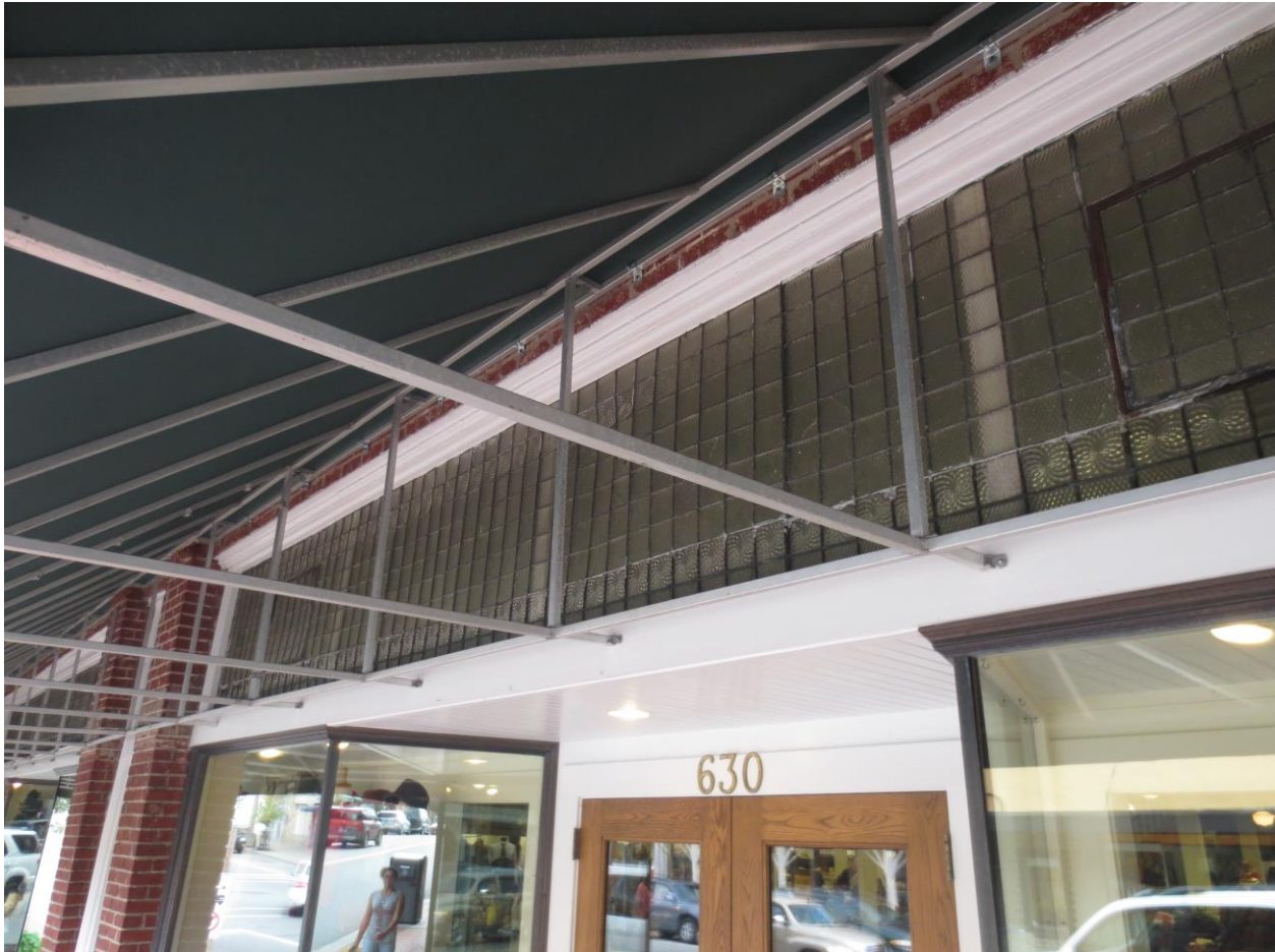
Original clerestory windows, like these found on one West King Street property, contain elaborate details that contribute to the character, appearance, and integrity of the downtown historic district. Photo courtesy of Eric Plaa, 2013.
