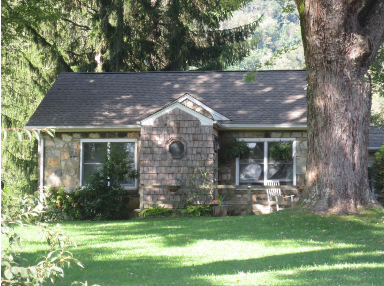
Original entrance configurations and porches should never be closed in or obscured by additions to historic properties, as has occurred with this otherwise attractive and significant Grand Boulevard home. Photo courtesy of Eric Plaag, 2013.
