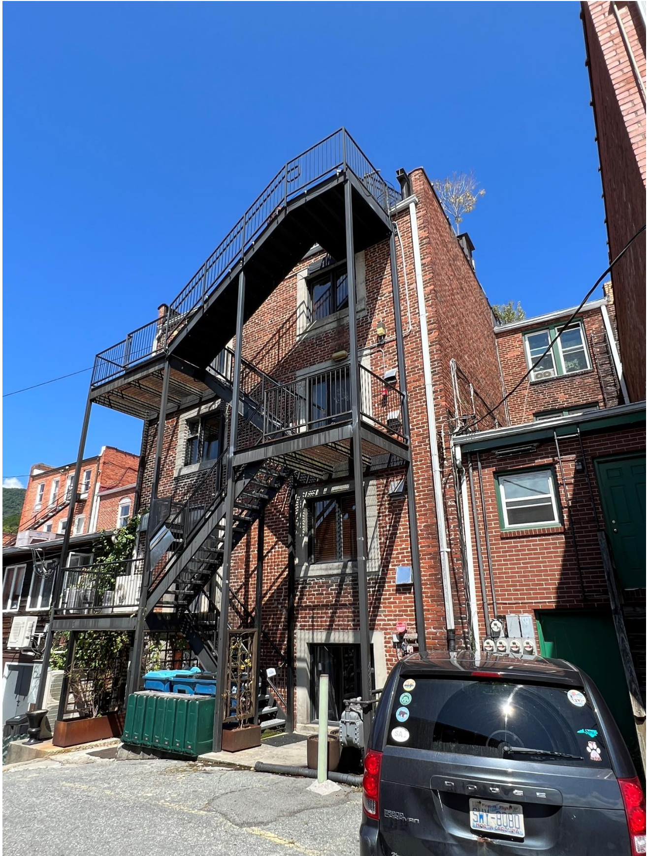
Communication: H.W. Horton Building Local Historic Landmark Designation - Current Images (H.W. Horton Building Local Historic Landmark
