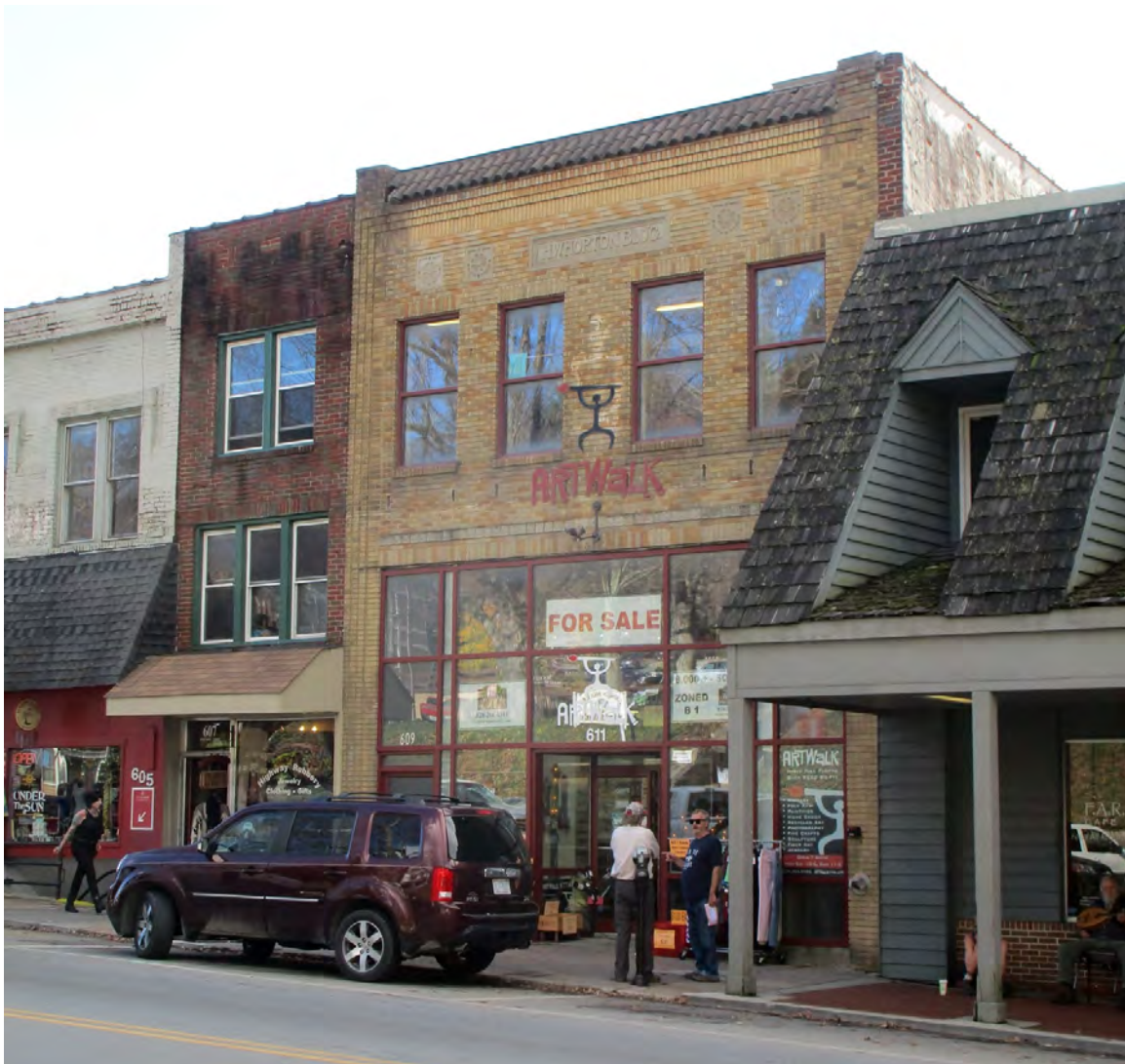
The H. W. Horton Building, November 2015. Image courtesy of Carolina Historical Consulting, LLC.
