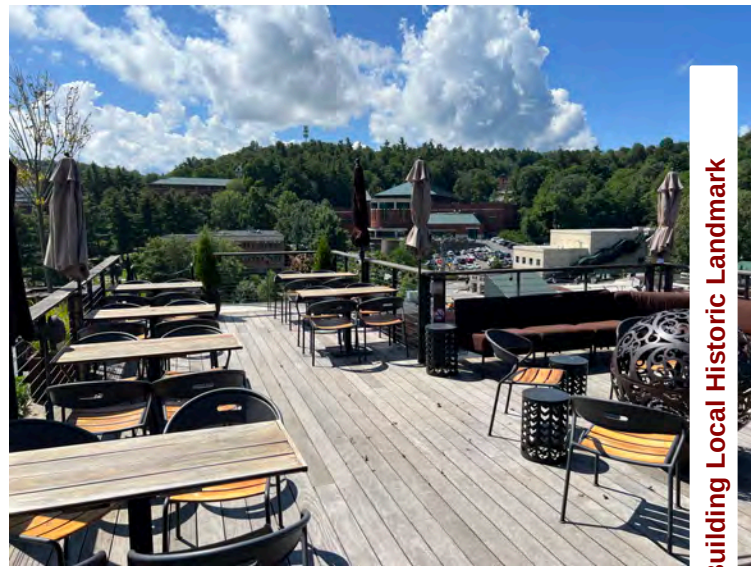
14. NC_WataugaCounty_HWHortonBuilding_0014.JPG H. W. Horton Building, rooftop deck rear, looking southwest
