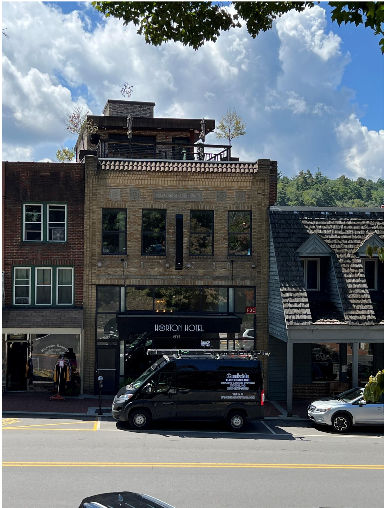
Communication: H.W. Horton Building Local Historic Landmark Designation - Current Images (H.W. Horton Building Local Historic Landmark
