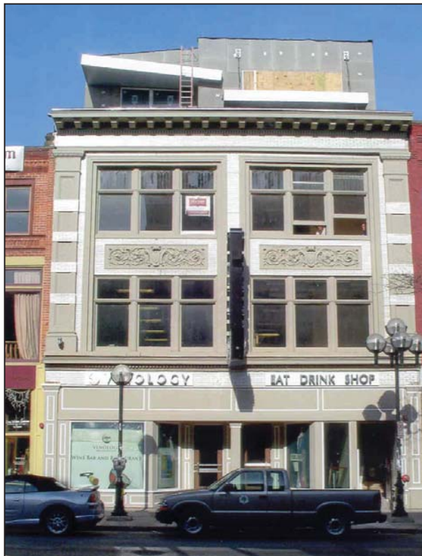
Three -story commercial building showing rooftop addition under construction.
