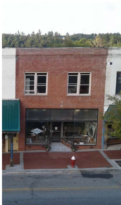
685 West King Street: Original brick materials, brick detailing; fenestration percentages; transoms; and storefront window
